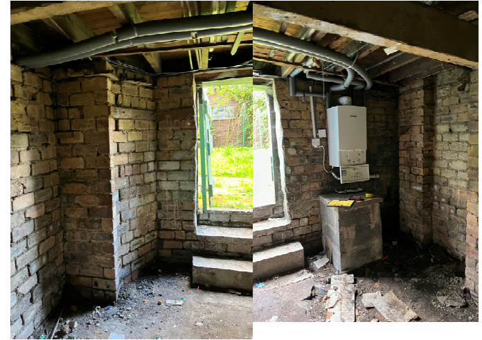
EXISTING BASEMENT VIEW
