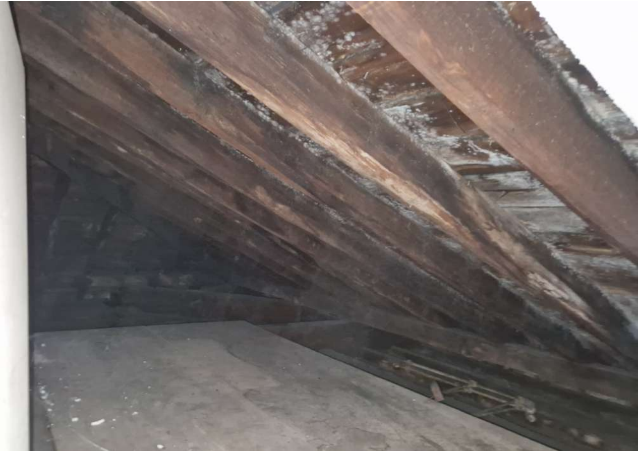
Existing roof joists to be demolished
