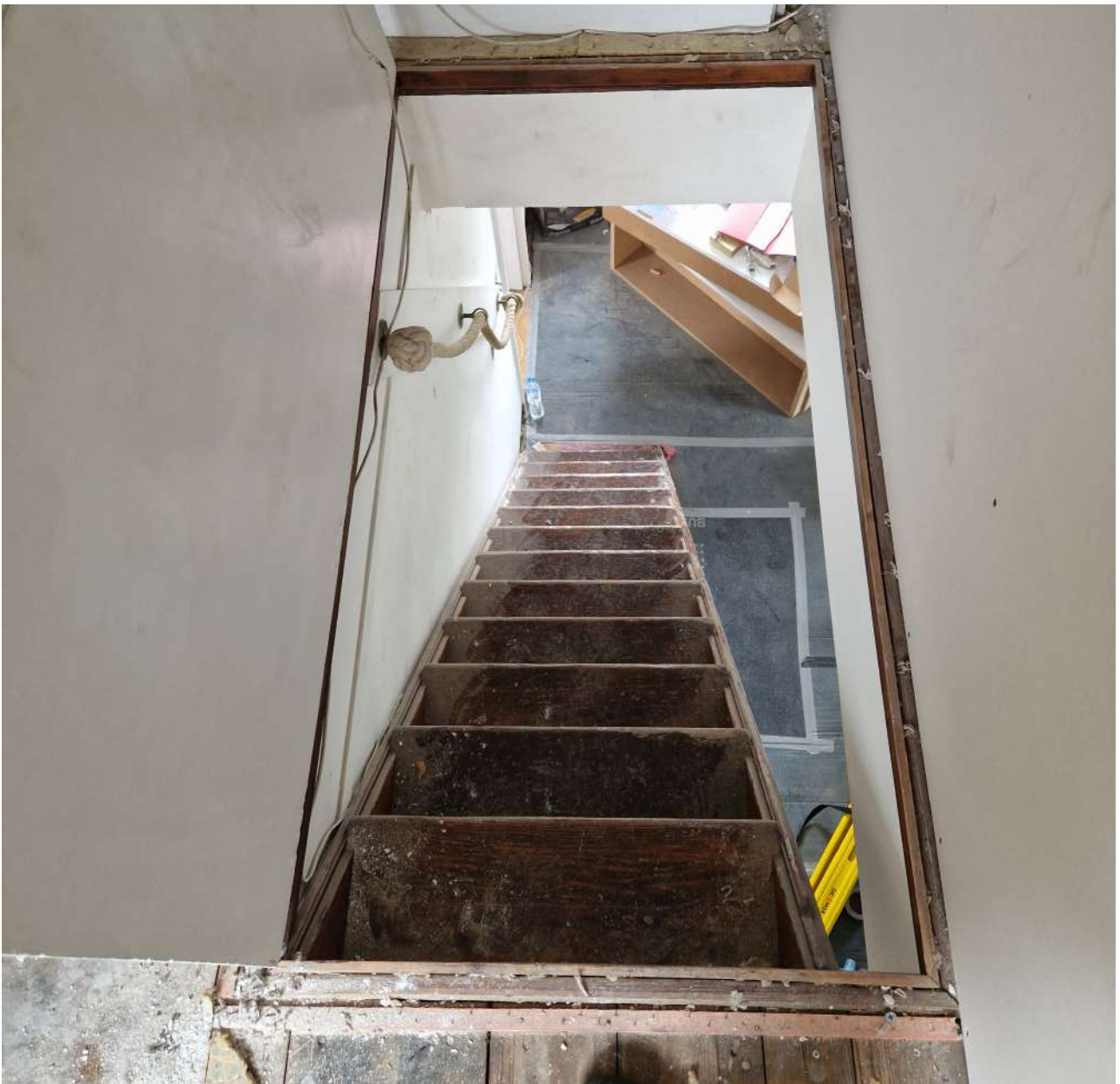
Existing staircase to loft.
