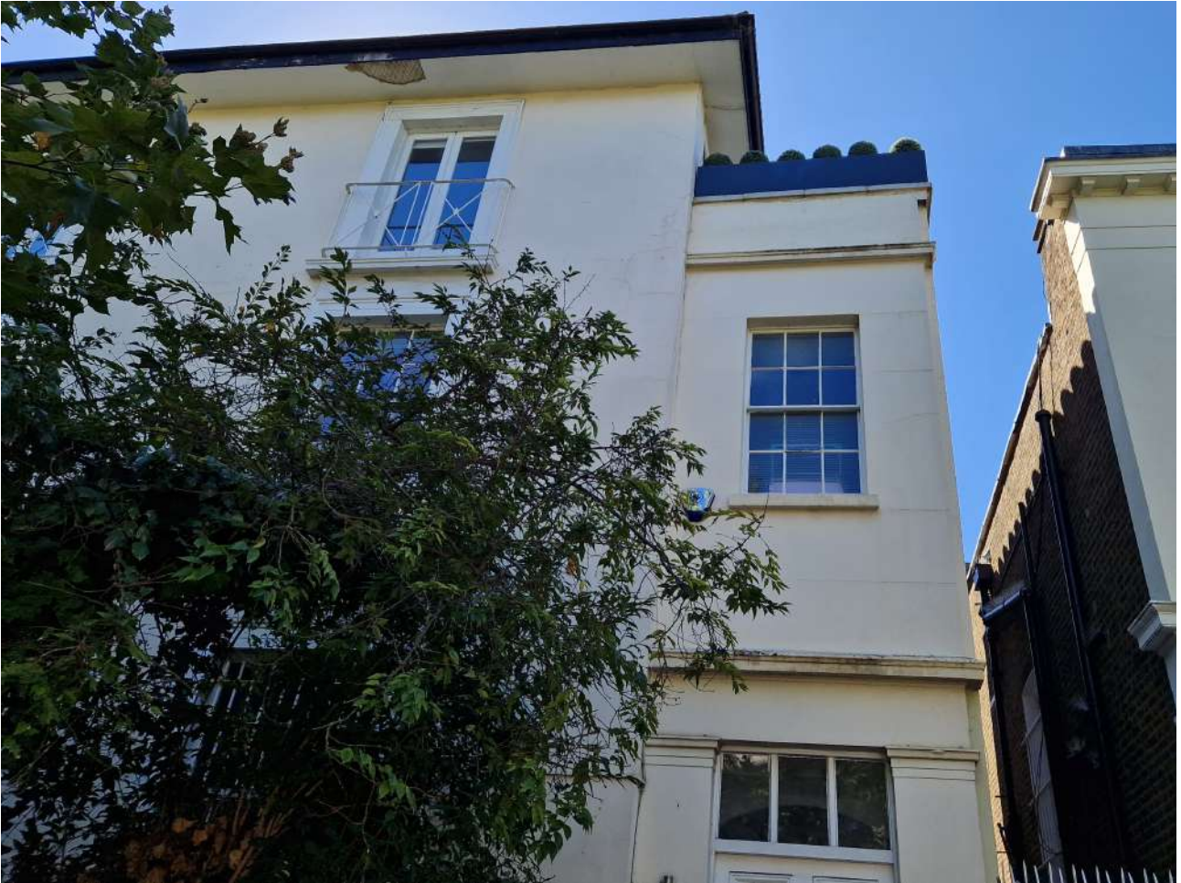
Existing stucco render - front facade.
