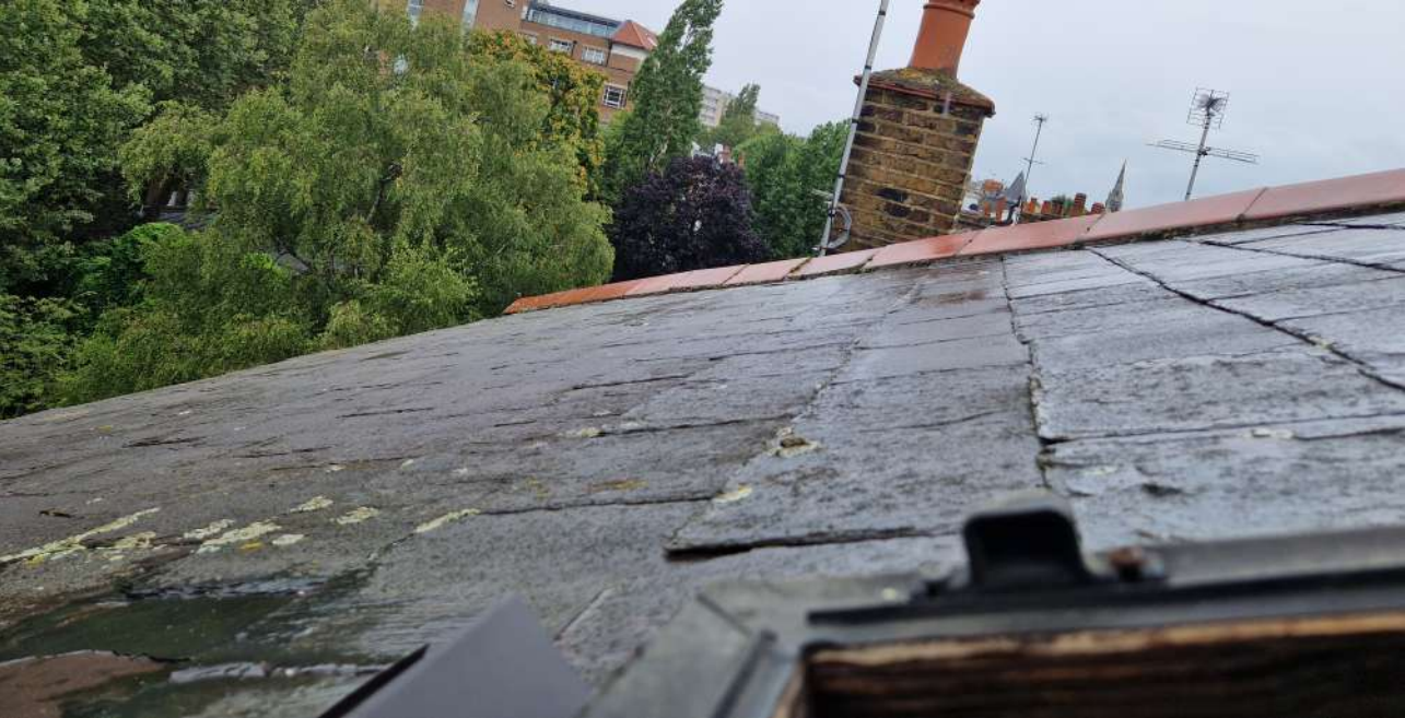
Existing slate roof tiles to be reused.
