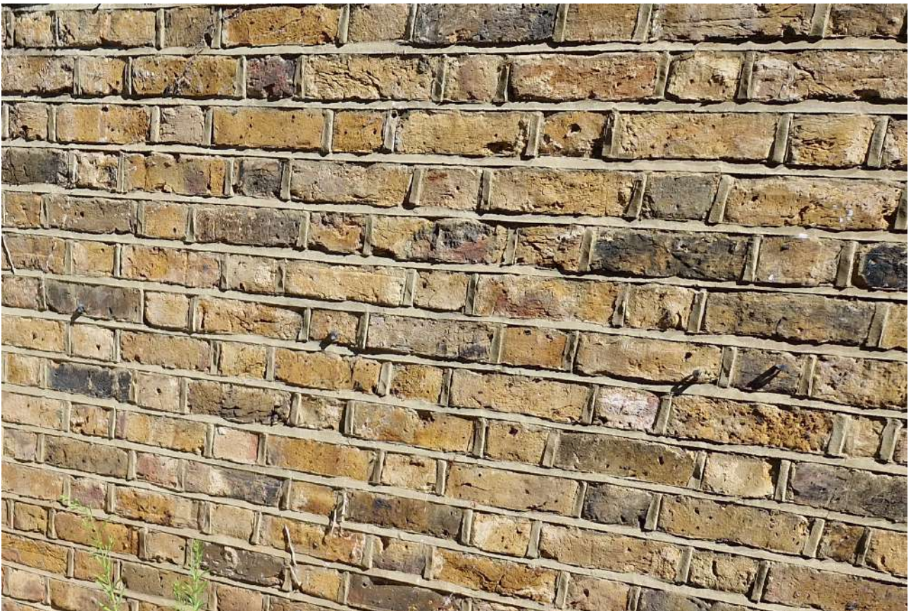
Existing yellow London stock bricks - rear and side facades.
