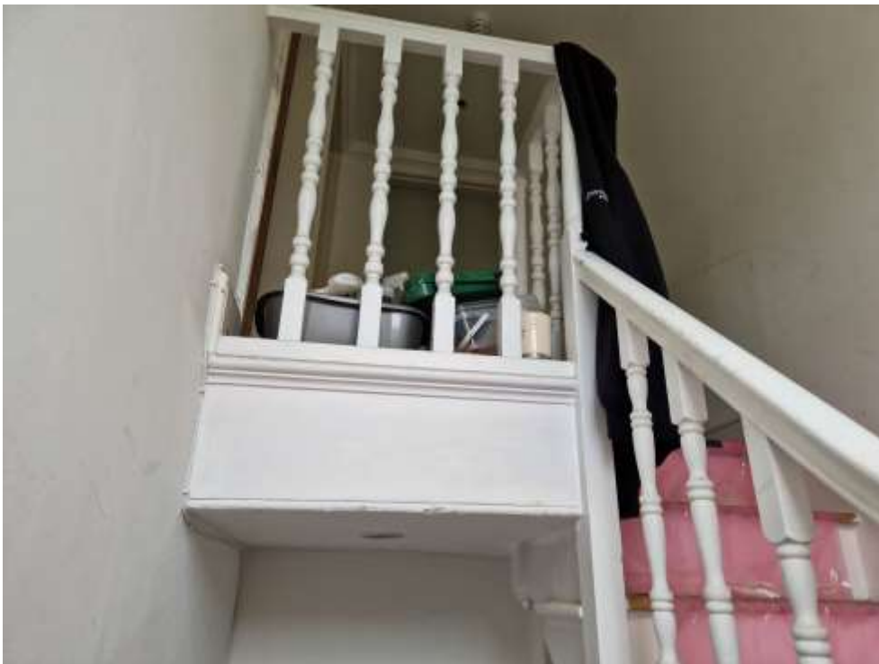
Figure 18 - View of the top floor landing, and the main stair balustrade.
