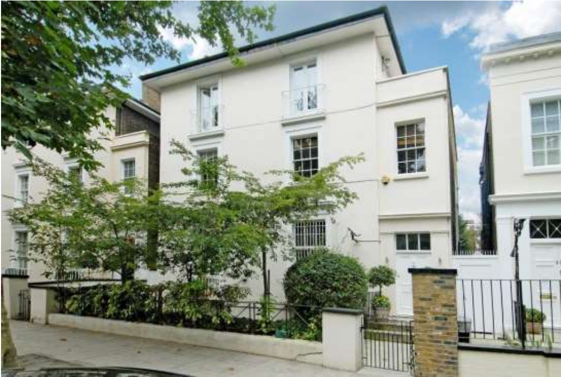
Figure 16 - View of the front elevation
