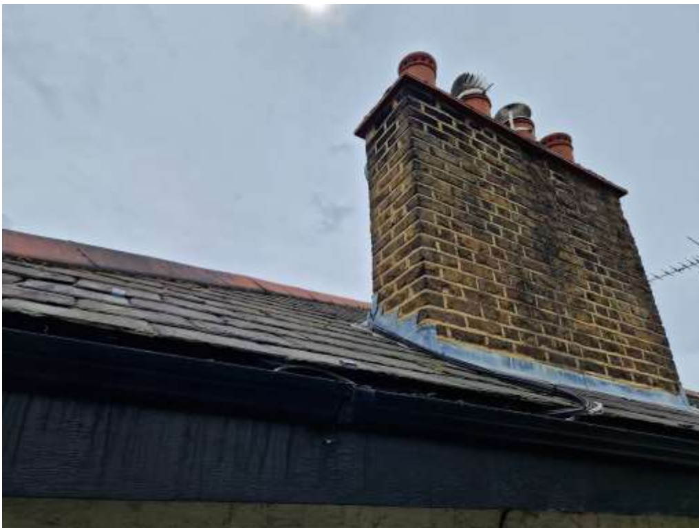
Figure 28 – View of the roof slate and the chimney stack.
