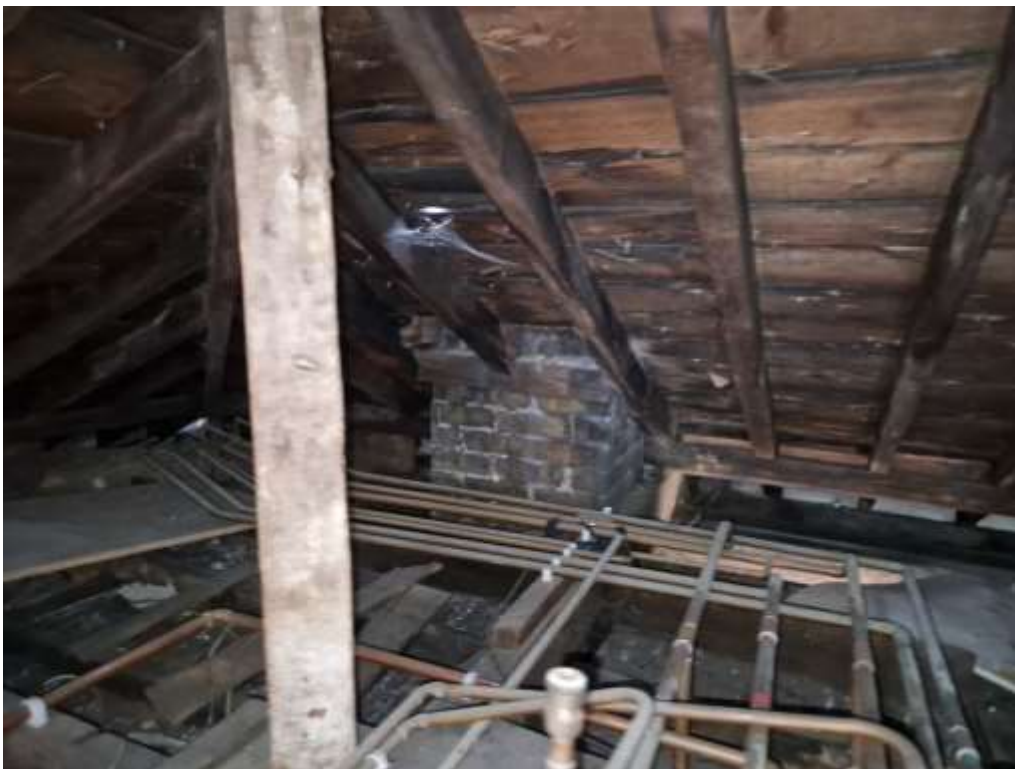
Figure 26 – View of the roof area behind the panels
