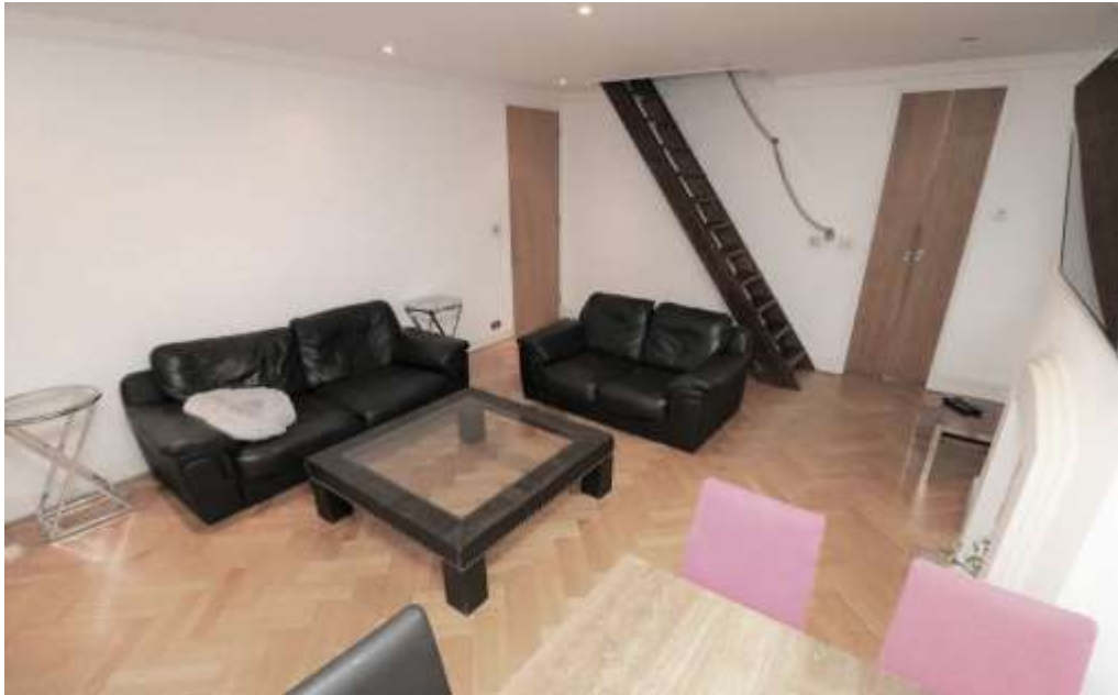
Figure 21 – View of the living room area, showing modern doors, stairs to the attic, and modern fire surround. Ceiling has spotlights throughout. Coving is modern. Modern timber floor, in herringbone pattern.
