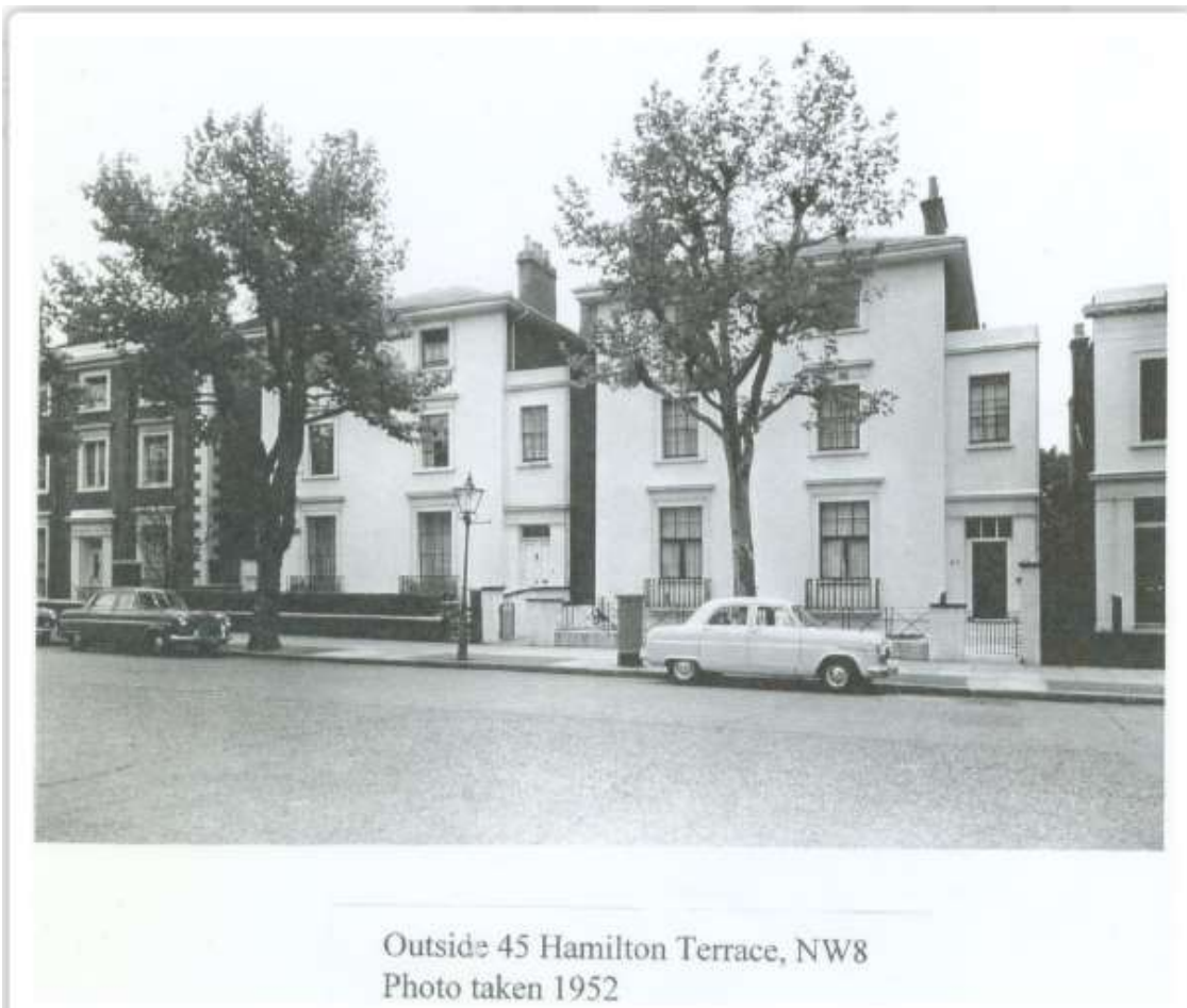
Figure 13 – 1950s photograph of the subject site (building to the right)
