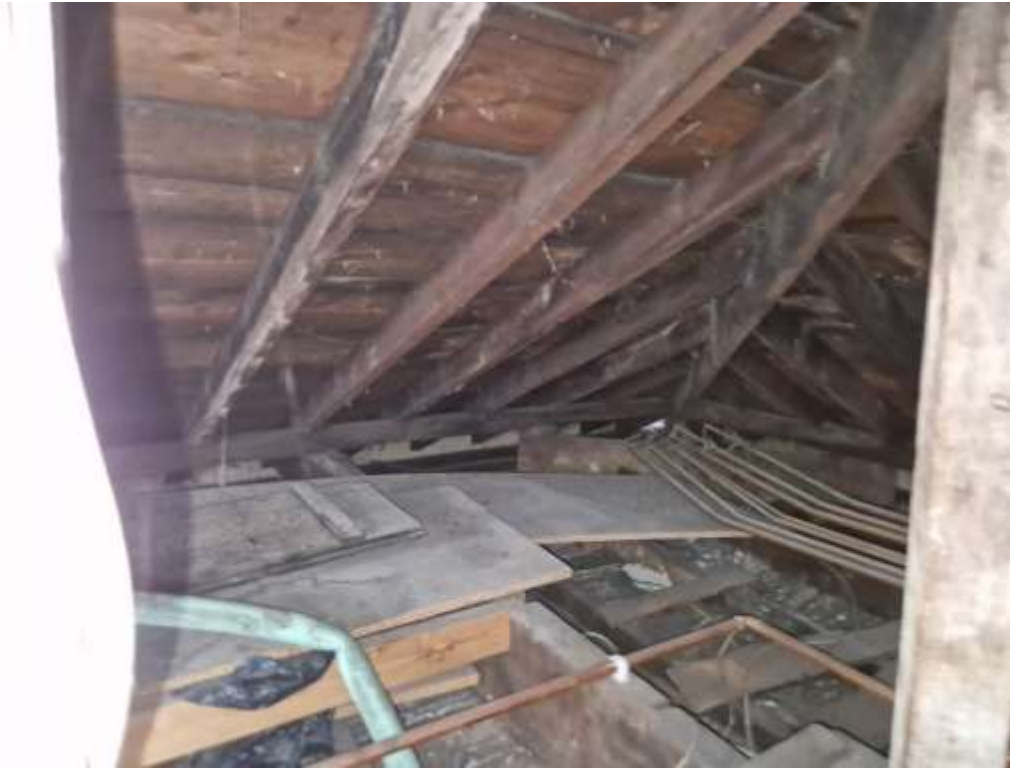
Figure 27 – View of the roof rafters with sarking boards over.
