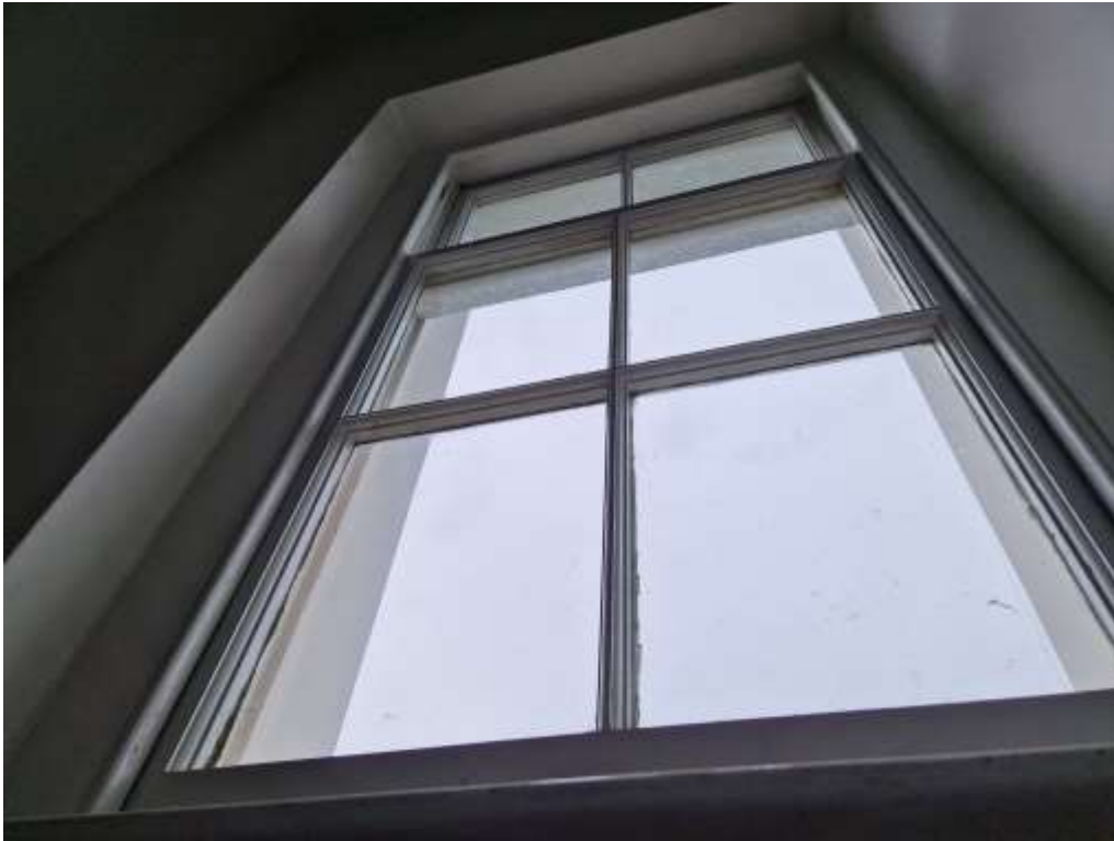
Figure 19 – Window to the stairwell.
