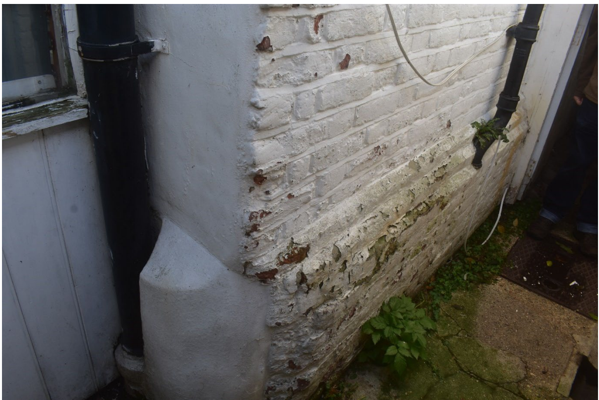
Figure 7. Turning corner for the former carriageway on the rear wall of 58 St Dunstan's Street.
