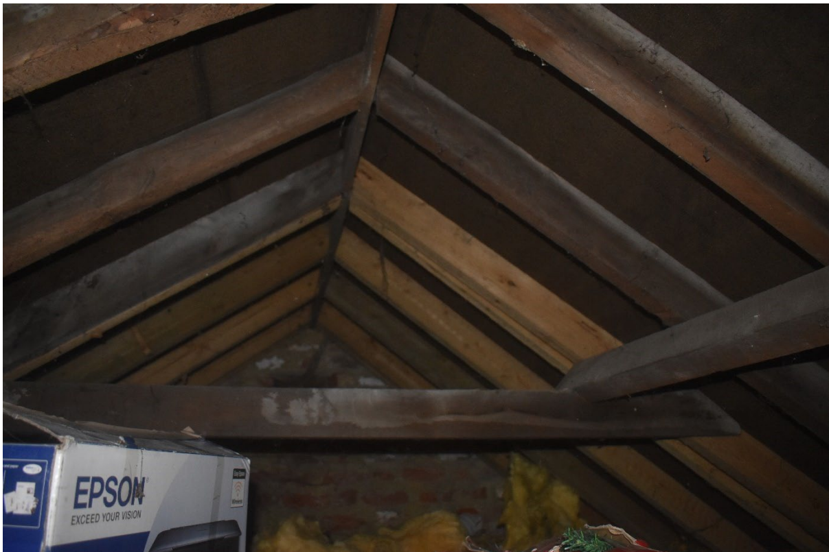
Figure 28. Modern rebuild of the rear outbuilding: machine sawn timbers and ridge board.
