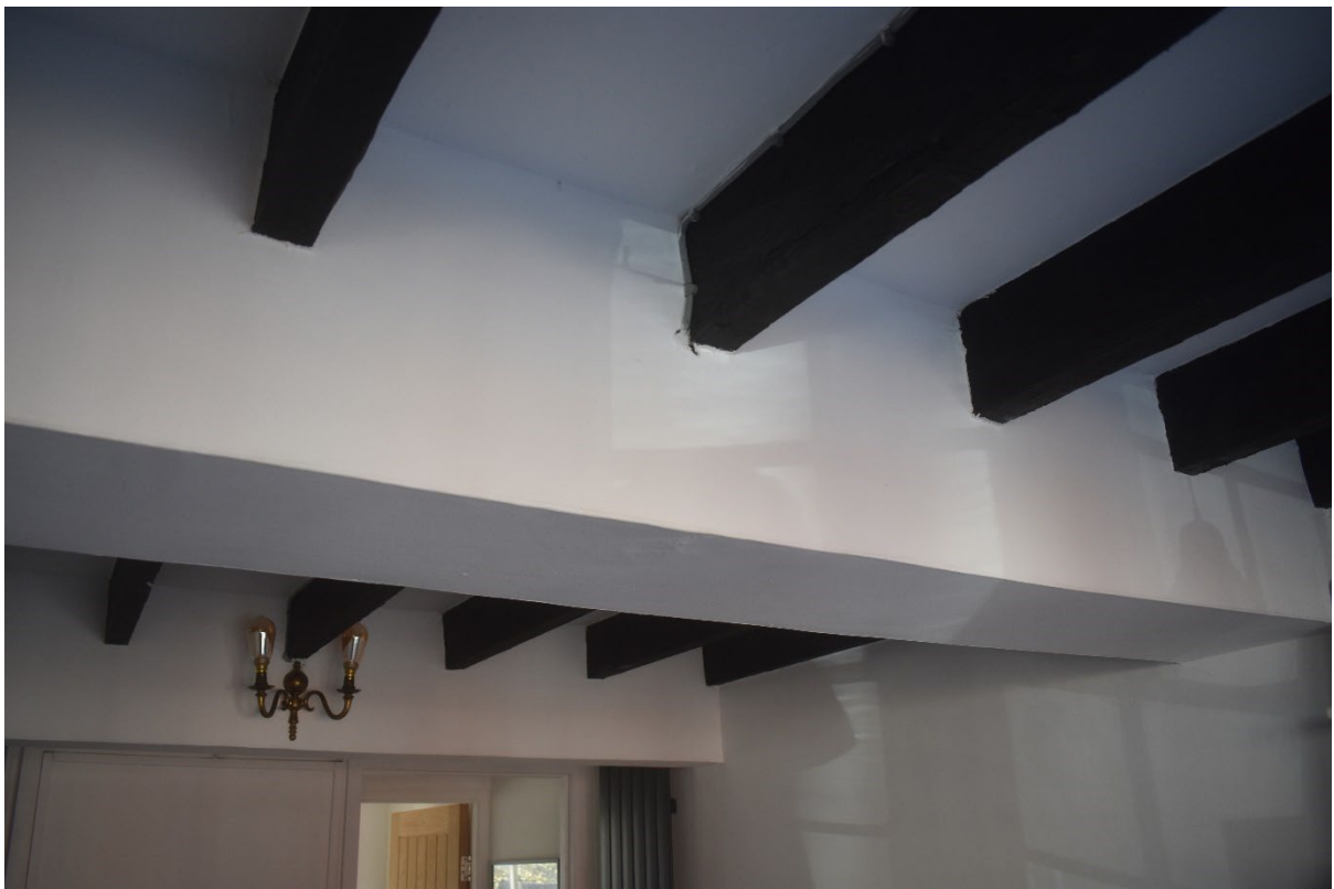
Figure 14. 59 Boxed in earlier timber framing on the first floor
