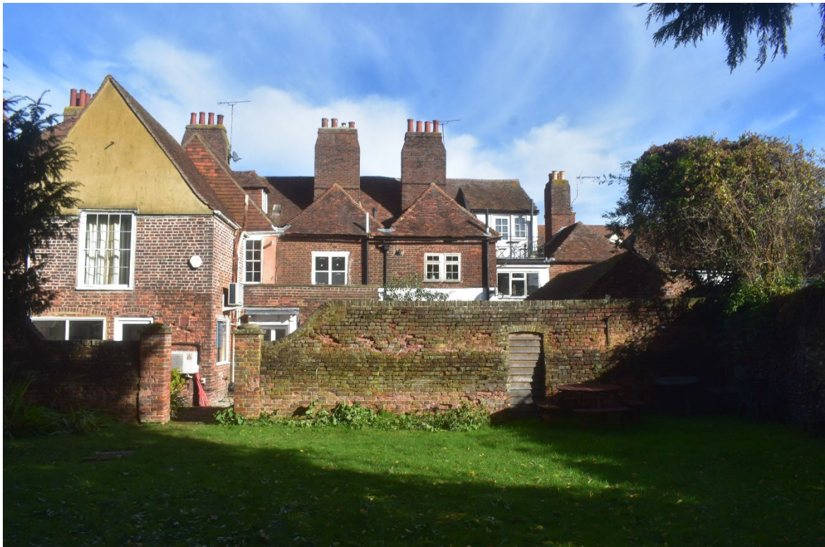
Figure 2. 59 St Dunstan's Street, in the context of the group of buildings, looking north-east
