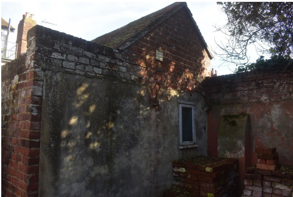
Figure 23. Late Victorian (?) gable at the south-west end of the rear outbuilding.
