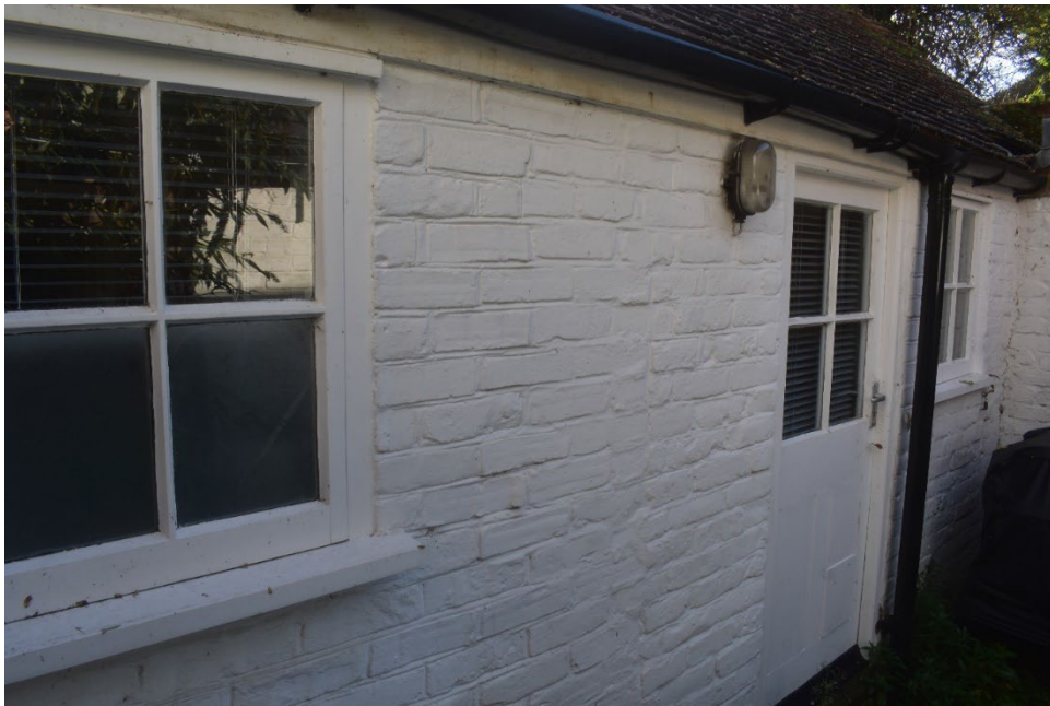
Figure 25. Modern rebuild of the rear outbuilding
