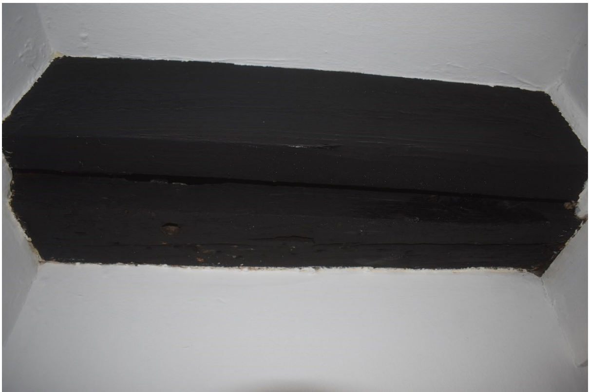
Figure 16. Detail of earlier reclaimed timber frame abutted by later
