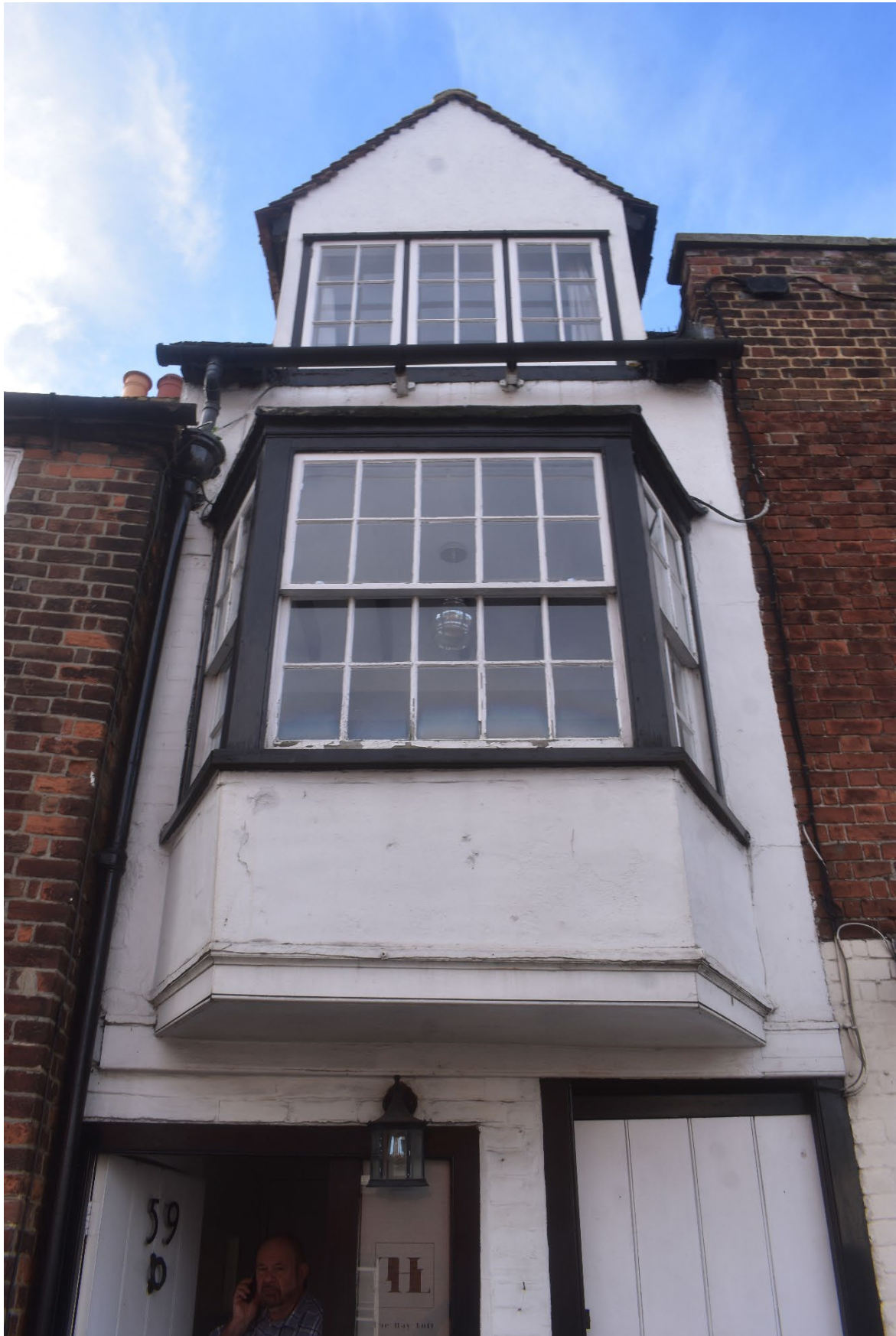
Figure 21. The nineteenth-century oriel/bay window, with later dormer above
