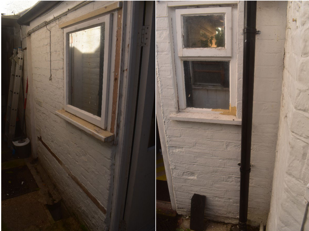
Figure 26–7. Modern rebuild of the rear outbuilding
