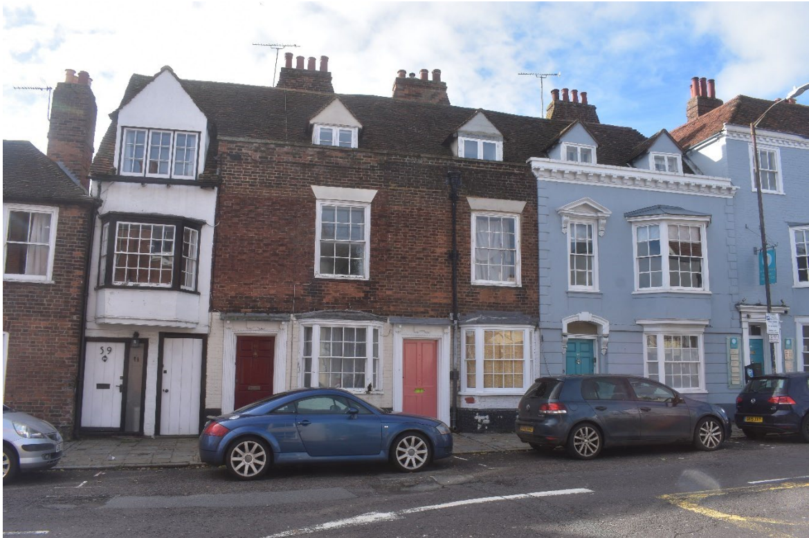
Figure 1. 59 St Dunstan's Street, in the context of the group of buildings, looking south-west
