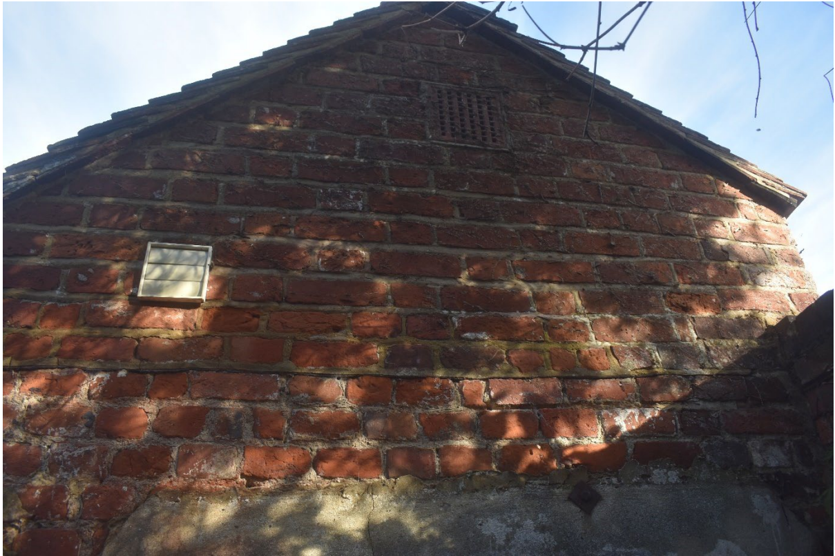
Figure 24. Late Victorian (?) gable at the south-west end of the rear outbuilding, noting the change of bond from English to Flemish, and also introduction of machine made bricks and vent.
