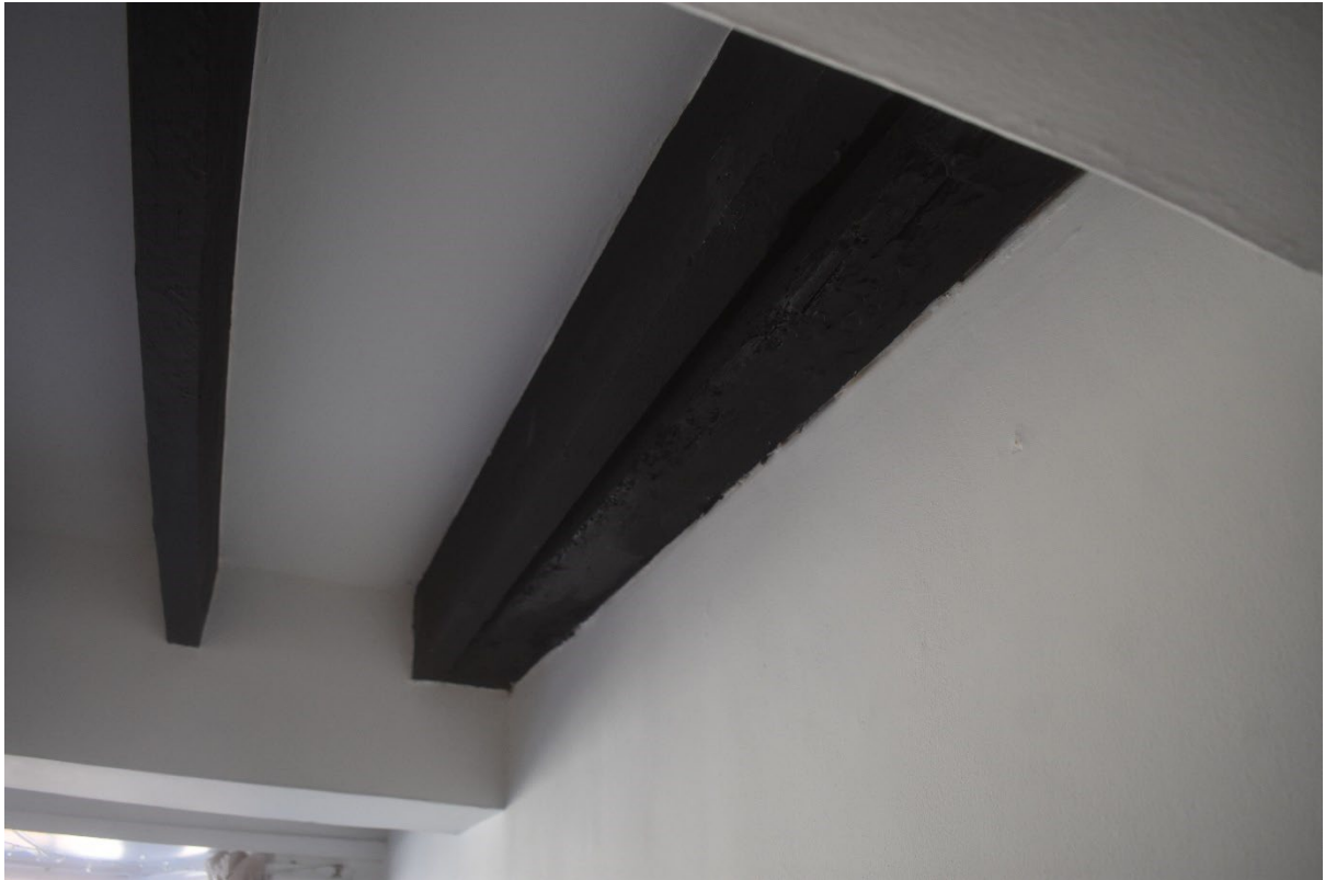
Figure 15. Earlier reclaimed timber frame abutted by later
