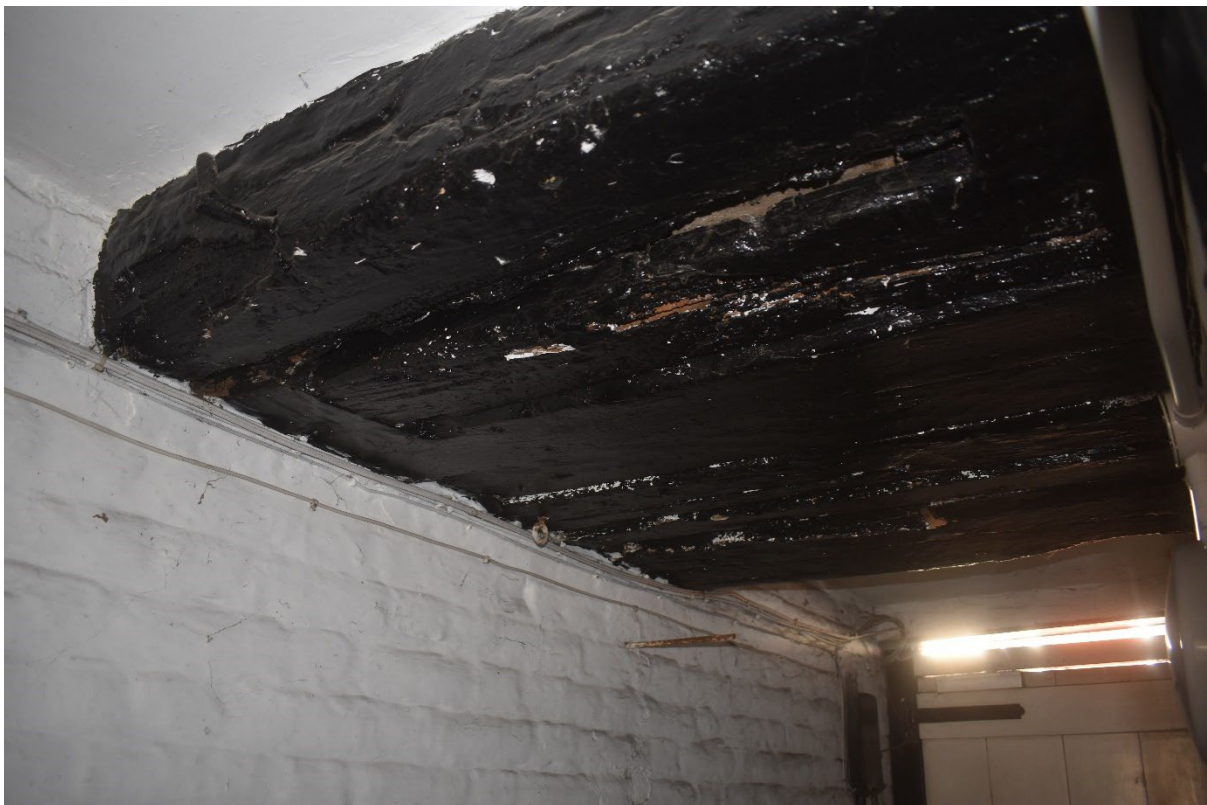
Figure 12. Reclaimed timber to form the first floor of 59 St Dunstan's Street, also suggesting some industrial use.
