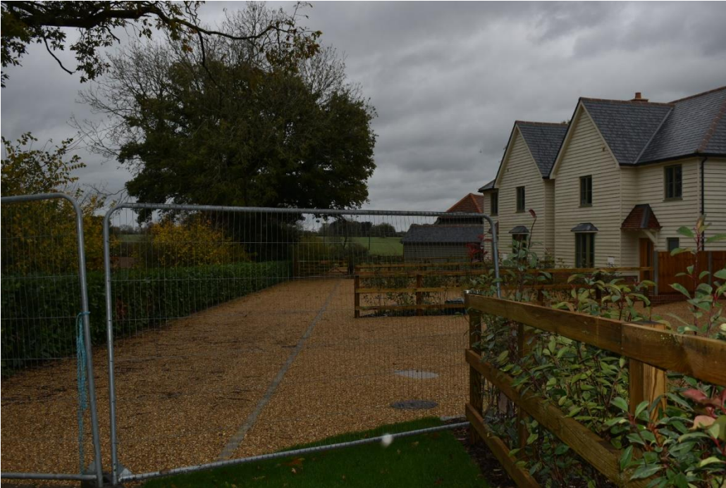
Photo 1 – new housing and access near completion
