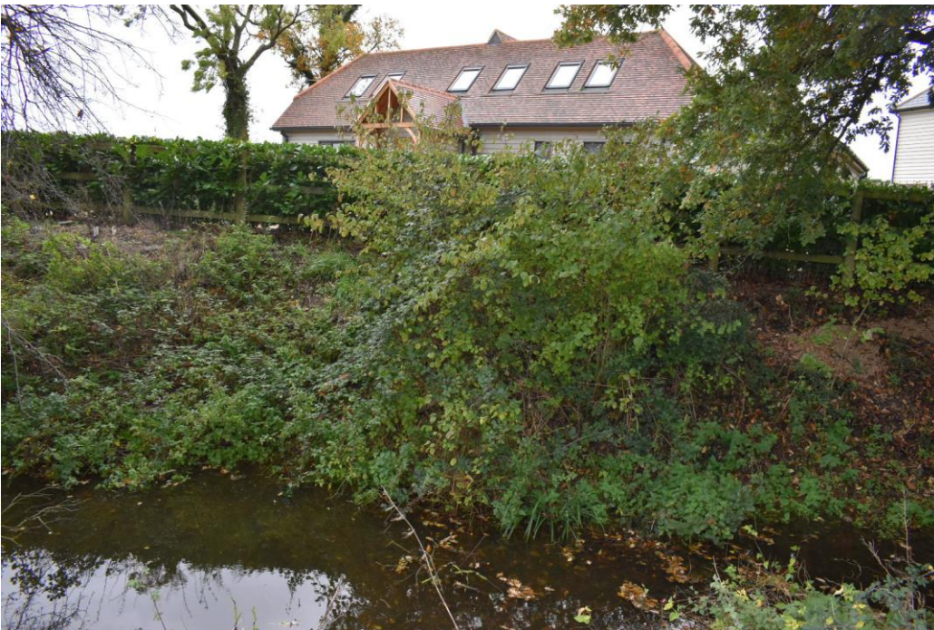
Photo 2 – new development extends to the top of the pond bank
