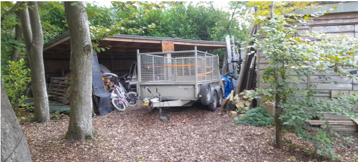
Existing South West Elevation of Covered Shelter
