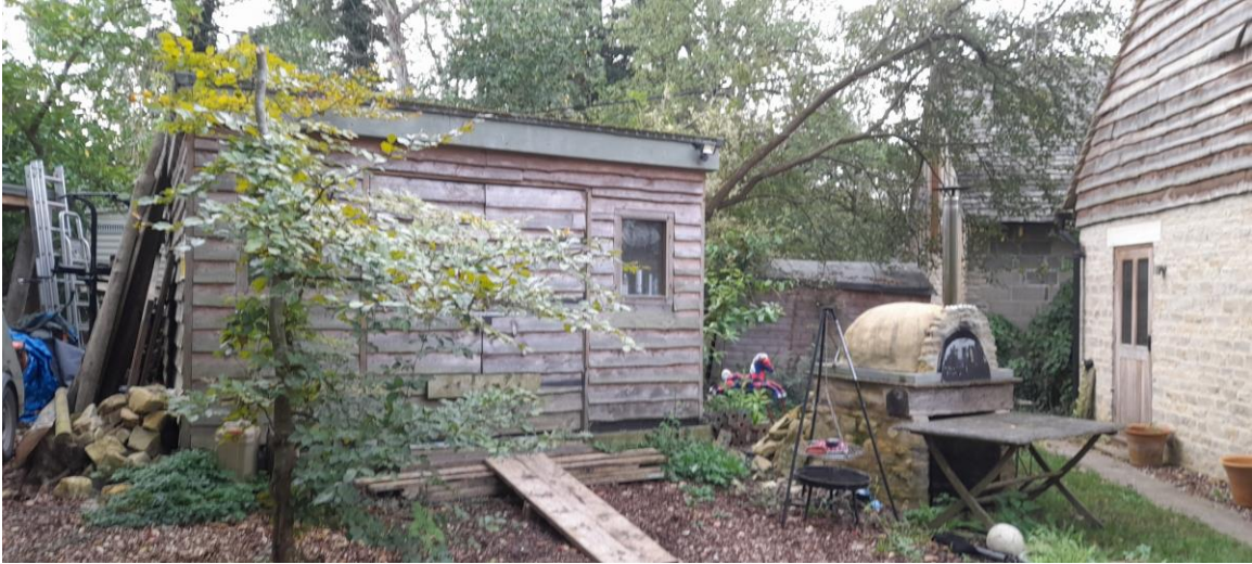
Existing North West Elevation of Shed
