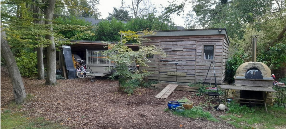
Existing North West Elevation of Shed
