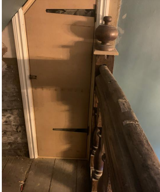
Figure 16. New access into loft area, previously an open space.
