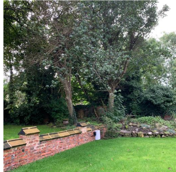
Figure 26 garden wall with repairs to copings and electrical box installed.
