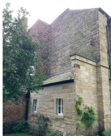
Figure 9 North elevation of the Vicarage showing the record room which contains a safe
