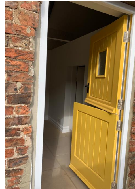
Figure 22 New external door to utility area
