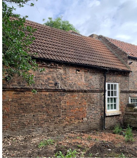
Figure 29 Church Road elevation of out building showing changes to openings.
