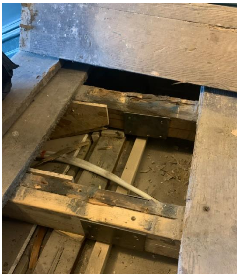
Figure 10 showing steel plates and new timber to support existing historic timbers.
