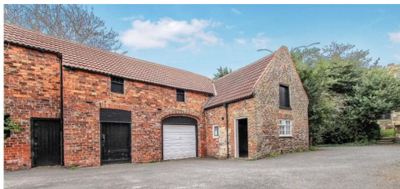
Figure 27 Existing outbuilding viewed from the east front of the Vicarage.
