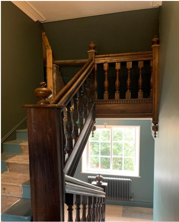
Figure 14 Existing staircase at attic level
