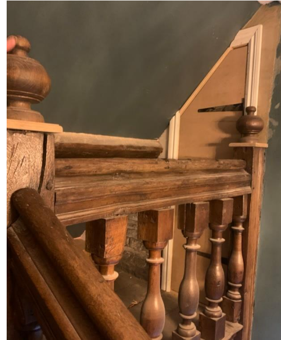
Figure 15 Historic stair details with minor oak repairs
