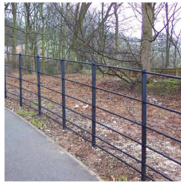
Steel estate fence painted black
