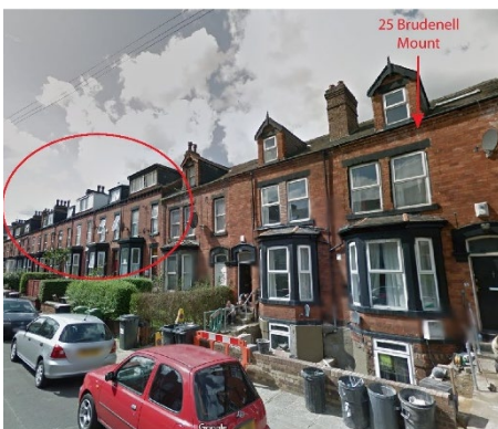
Picture 1: Existing dormers across Brudenell Mount.
