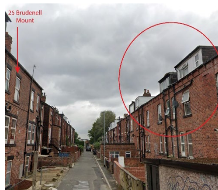
Picture 2: Existing dormers on Back Brudenell Mount.
