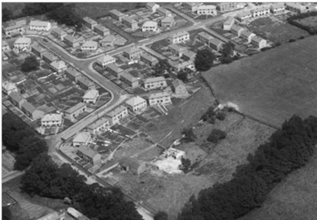
Plate 2: Circa 1926 aerial photograph showing the remains of the building platform of the Hall and retained agricultural building fronting onto Carr Road (Historic England: EPW016216).
