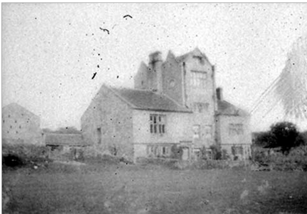
Plate 1: Newall Old Hall following partial demolition and reconstruction. Circa 1900. ( http://www.leodis.net/display.aspx?resourceid=20041025_80202884&DISPLAY )
