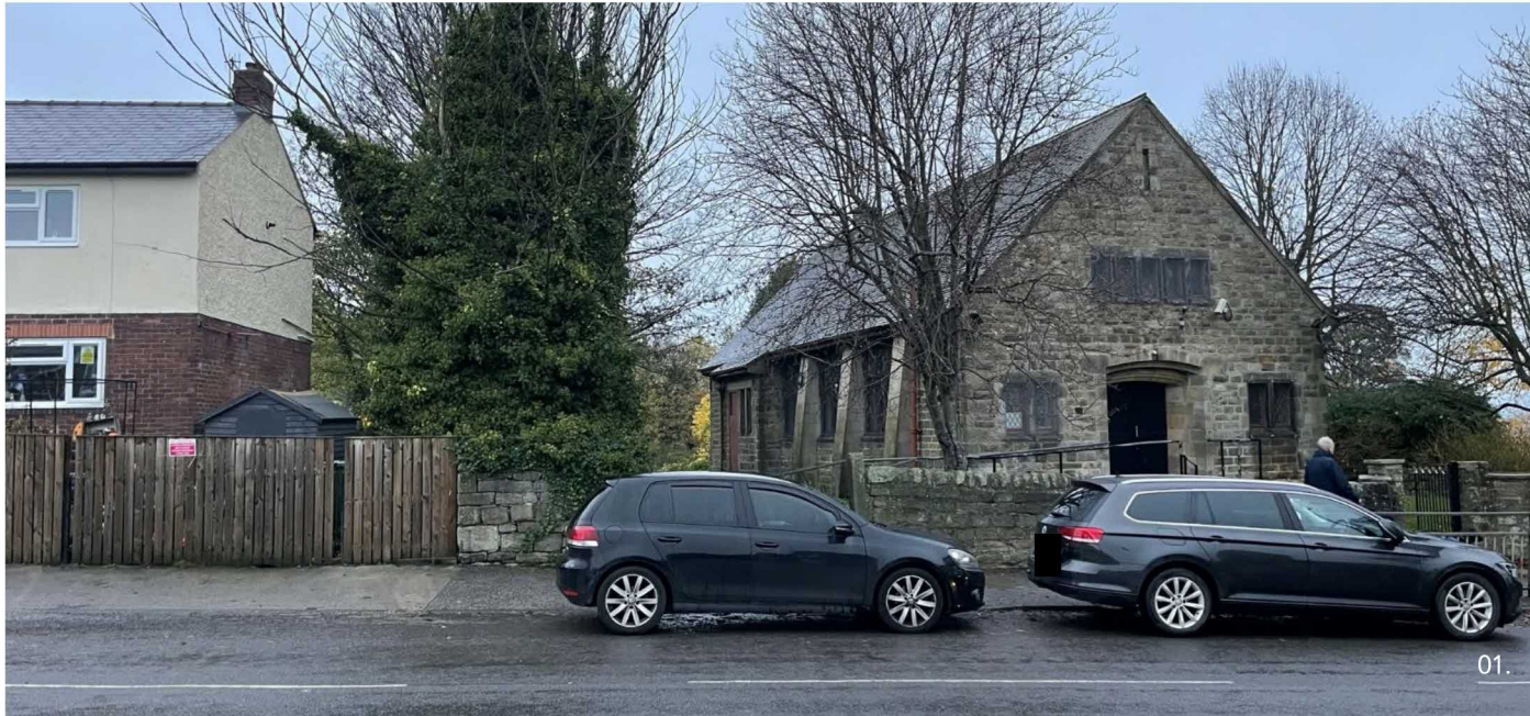
No. 01 – View of the redundant Church Hall from Newall Carr Road.
