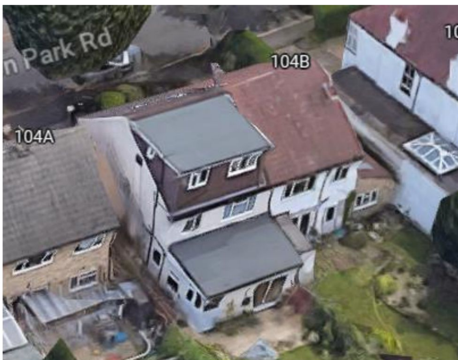
Aerial view of 104 Carshalton Park Road, showing large rear dormer
