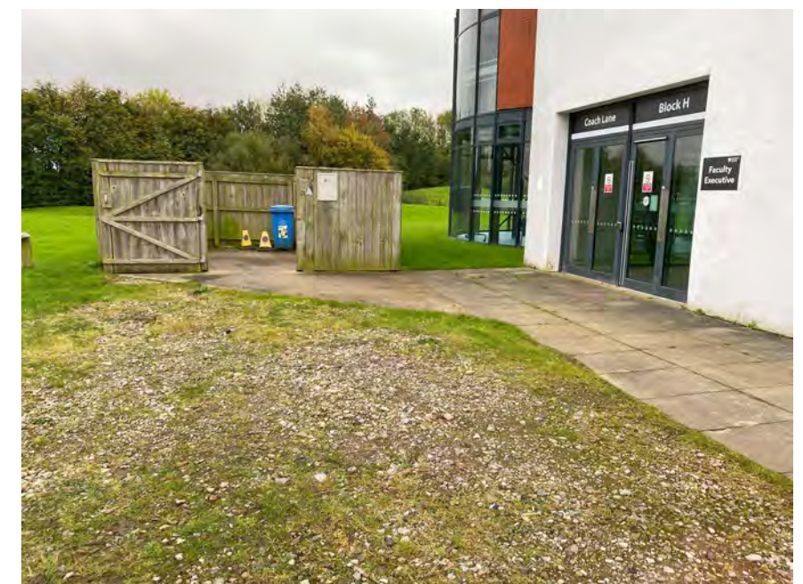
Fig 9: ASHP Location – External Compound
