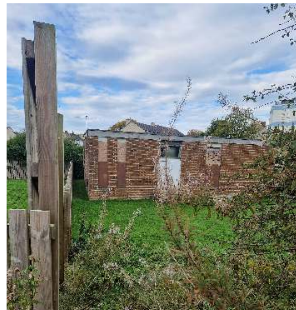
3. Street View - from Mungo Park
