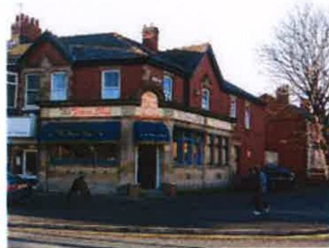
Fig. 18 Former bank at junction of Leamington Road and Whitegate Drive
