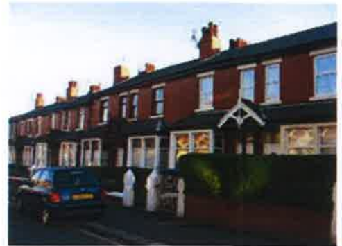
Fig. 36 Typical terrace, Leeds Road
