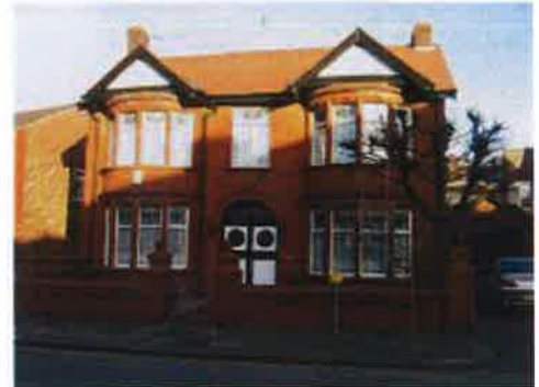
Fig. 38 29-31 Leicester Road: intact houses with possibly contemporary garage
