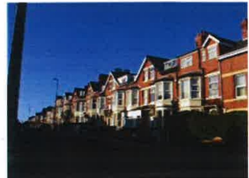
Fig. 34 Views up Hornby Road from the east
