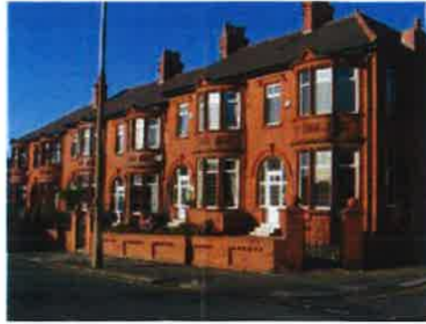
Fig. 46 Little altered, well detailed terrace (Nos. 32- 40) on the north side, built 1920s
