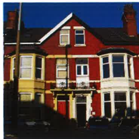
Fig. 20 Ironwork balconies and bay cresting (left) on Hornby Road
