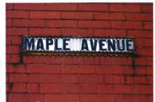
Fig. 19 Early 20th century street name signage, tiled letters in cast-iron frame
