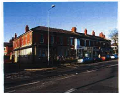
Fig. 39 1-13 including bank on junction with Leamington Road
