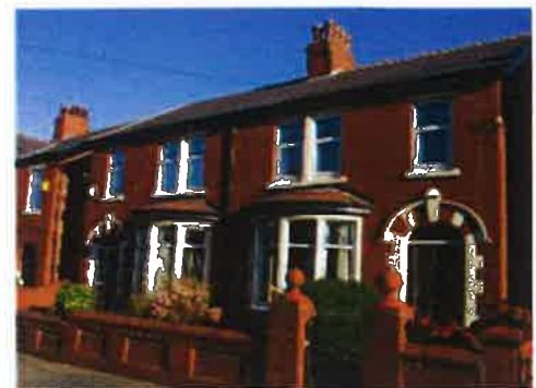
Fig. 22 Intact decorative brick boundary walls and gatepiers with terracotta details, Longton Road
