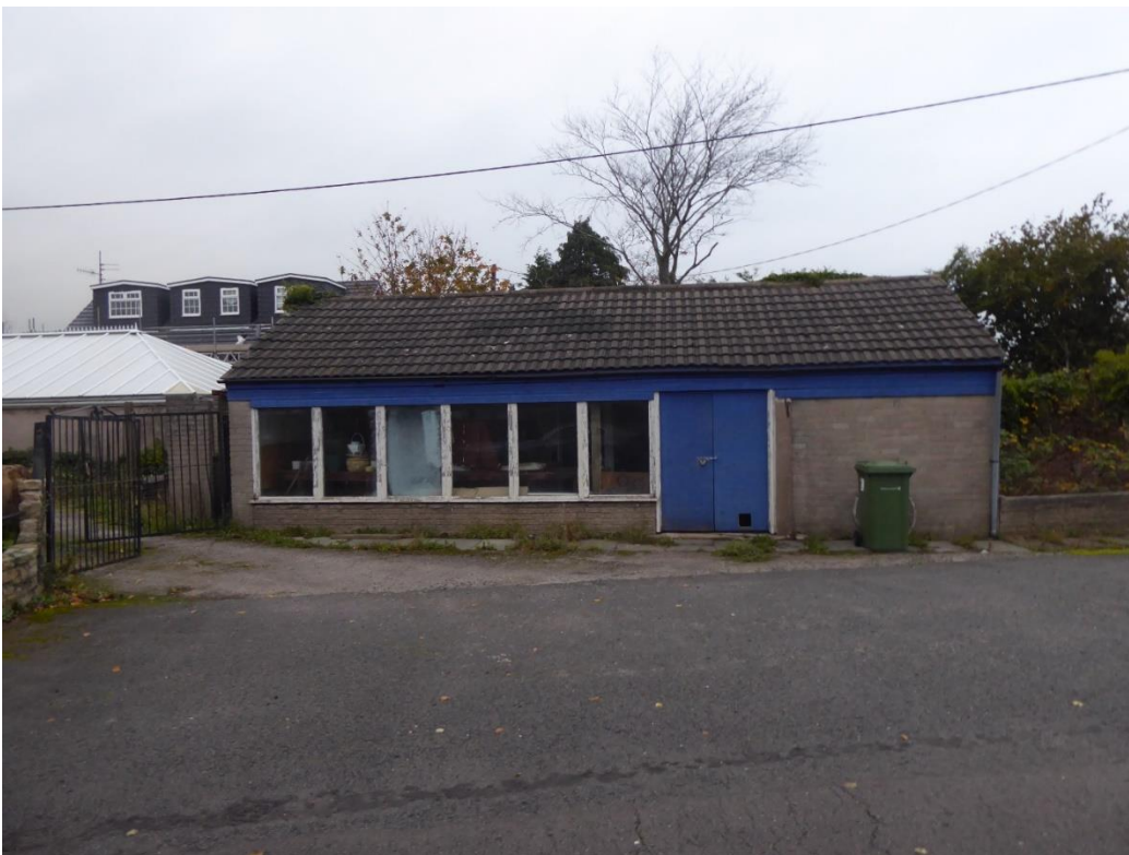
Photo 2 – Side Elevation of Garage
