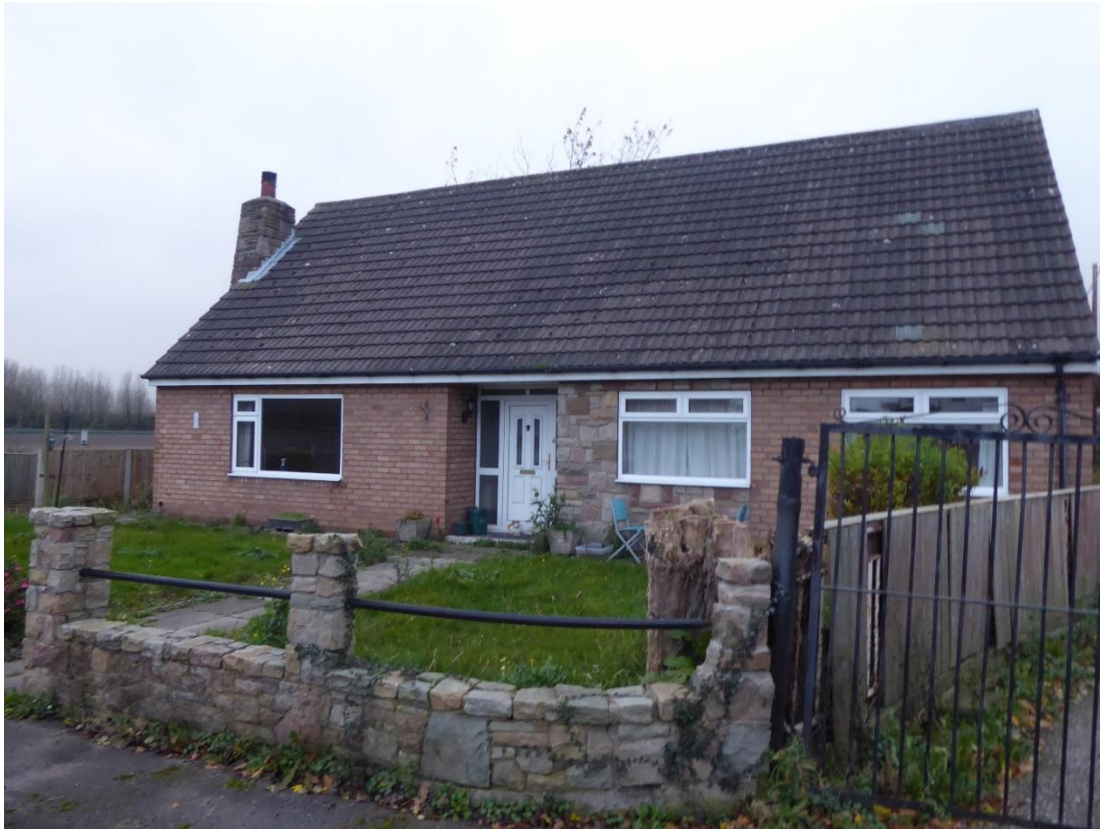
Photo 5 – Existing bungalow front elevation
