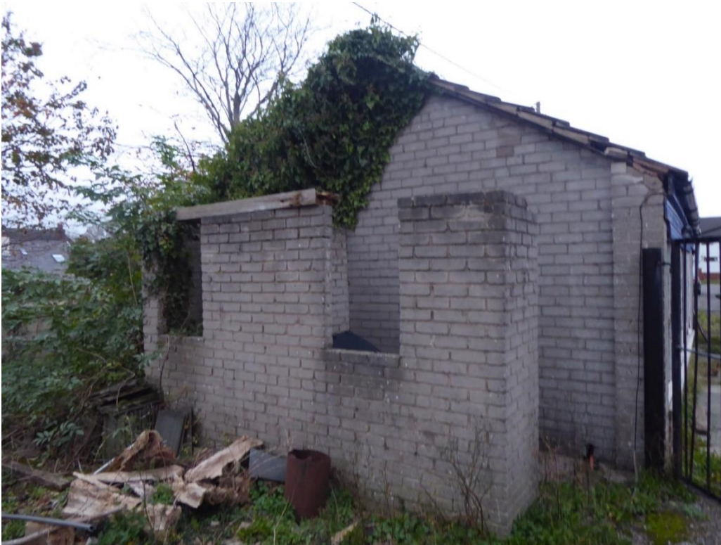
Photo 1 – Rear of detached garage
