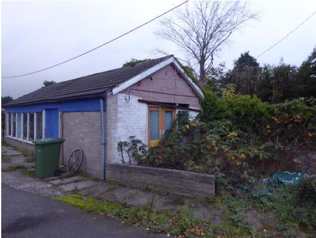
Photo 3 – Front elevation of Garage
