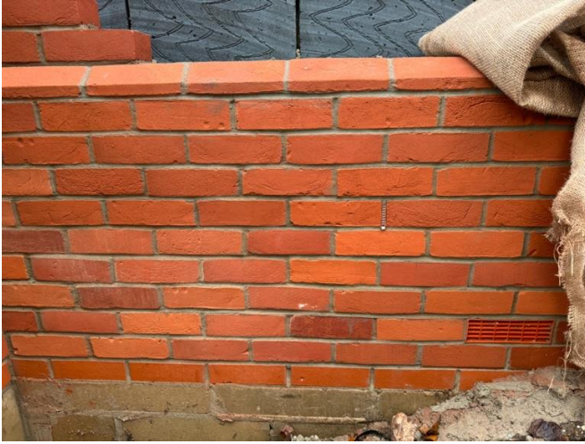
Sample mix of 3 sussex handmade clay brick , Waverly orange, Guestling red and Westfield
