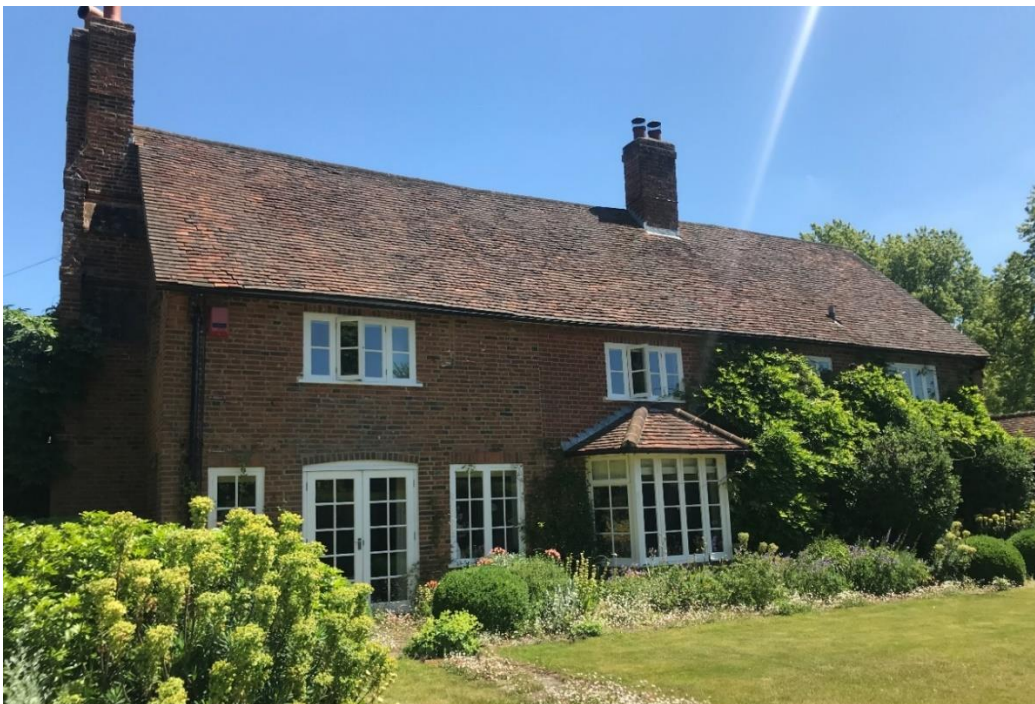
Figure 14: West elevation. The modern conservatory and pool room extension projects forward of the host building (right of image).
