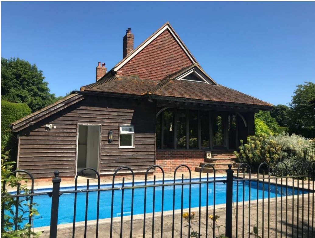
Figure 17: South end of the building, with modern conservatory and pool room extension behind the pool. The extension is overly dominant, with bulky roof form and footprint which extends significantly beyond the west building line of the host building (to left of the image).
