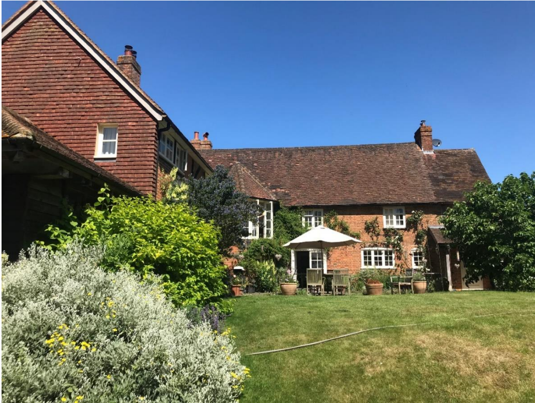
Figure 15: Looking north from the rear garden towards the house. The south gable end (left) is clad in modern tile hanging, with the modern conservatory extension projecting forward from it.
