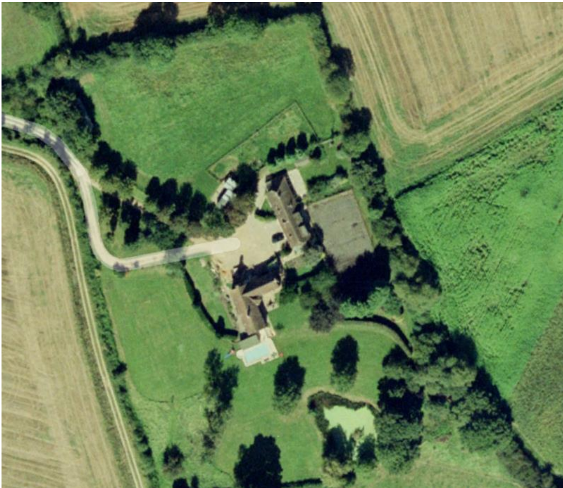
Figure 5: Aerial image, 1999. All earlier outbuildings now appear to have been demolished. The 'Cottage' has been built to the north-east of the main house, along with a tennis court appears to have been laid out to the east. The swimming pool and flat-roofed pool house is apparent at the south of the main house.
