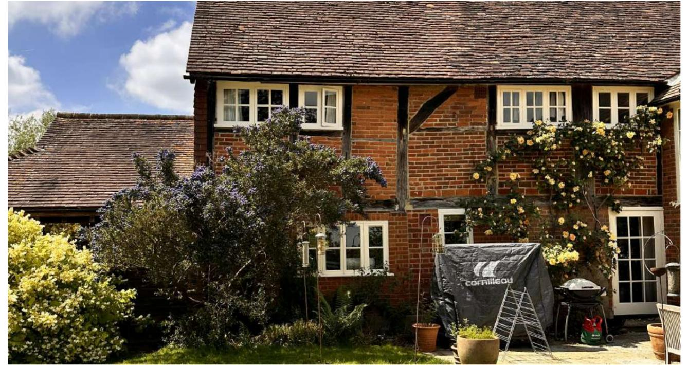
Fig.25: Existing post and beam with brick infill
