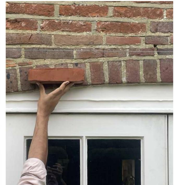
Fig.29: Brick survey pictures offering up a suggested brick against a variety of existing bricks from multiple elevations
