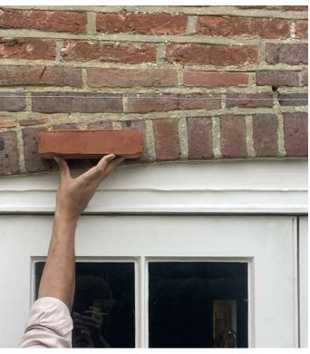
Fig.29: Brick survey pictures offering up a suggested brick against a variety of existing bricks from multiple elevations
