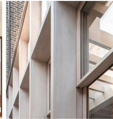
Fig.34: Untreated dried Oak frame and Windows
