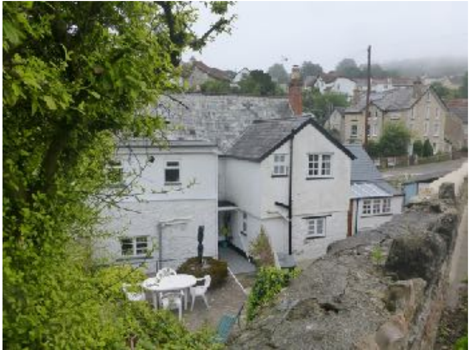
7. Highly visible two storey flat roof and pitched roof extensions on properties to the west of Wayside
