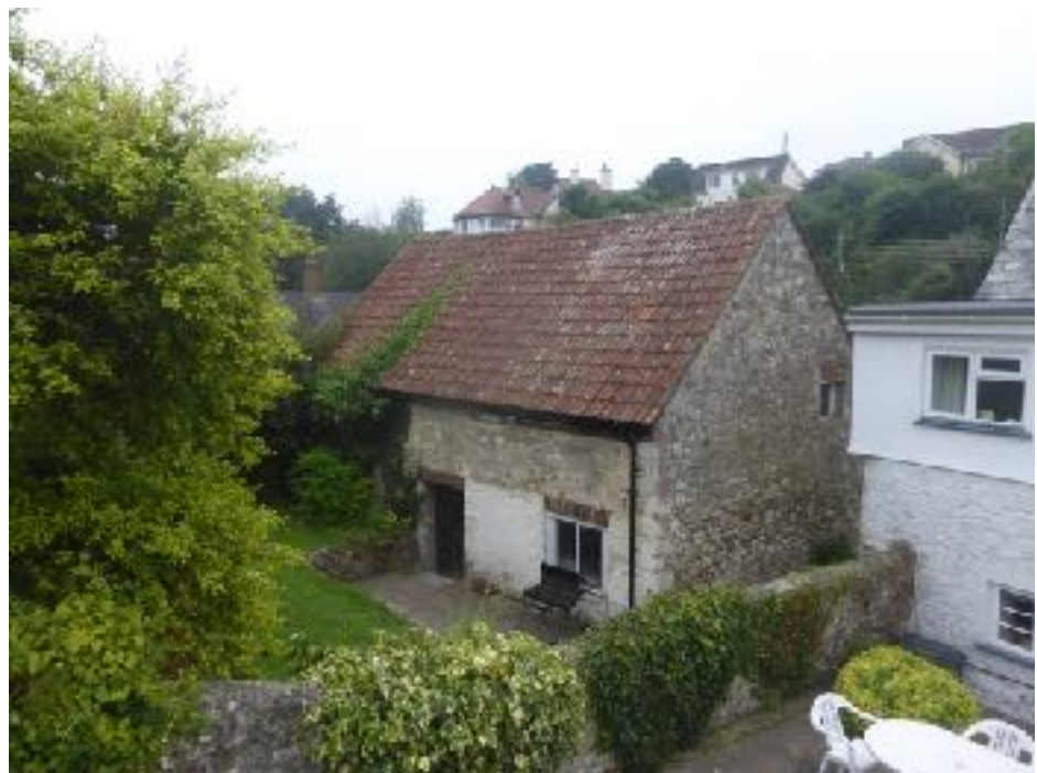
6. Rear elevation of Wayside is obscured by outbuilding and neighbouring concrete flat roof two storey extension
