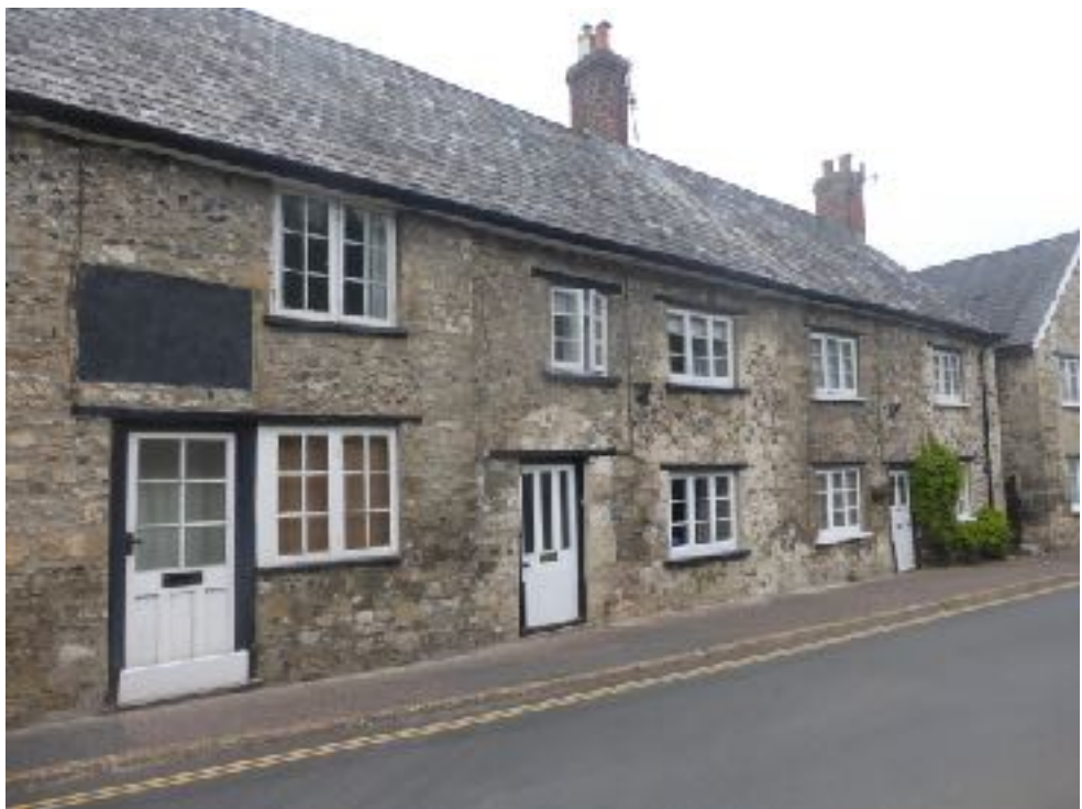
2. Wayside (on the left) in context of the rest of the terrace
