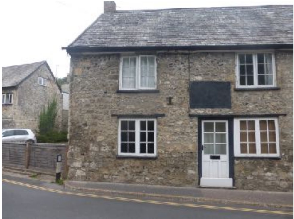
1. Front elevation of Wayside
