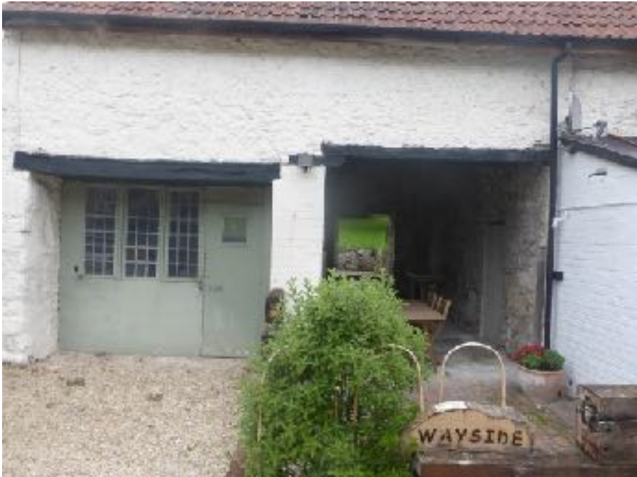
4. Front elevation of outbuilding to rear of Wayside
