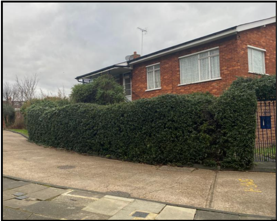
Image 2: Southern elevation of 19 Hertford Court (Source: surveyor photograph, June 2023)
