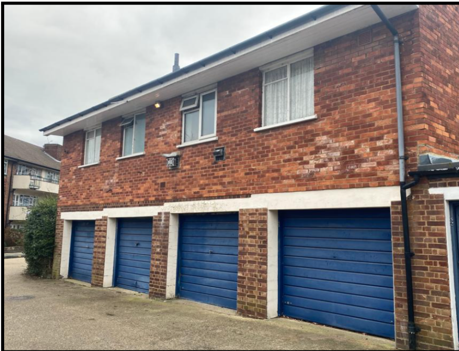
Image 1: Northern elevation of 19 Hertford Court (Source: surveyor photograph, June 2023).
