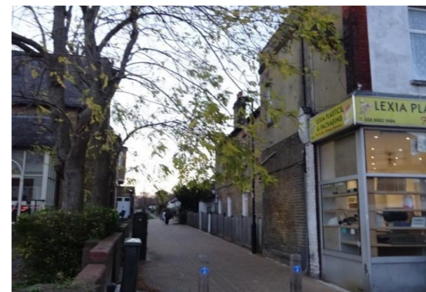
IMAGE 13: the existing buildings seen from Green Lanes.
