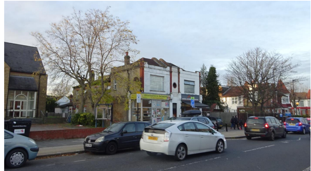
IMAGE 1: Existing building seen from Green Lanes
