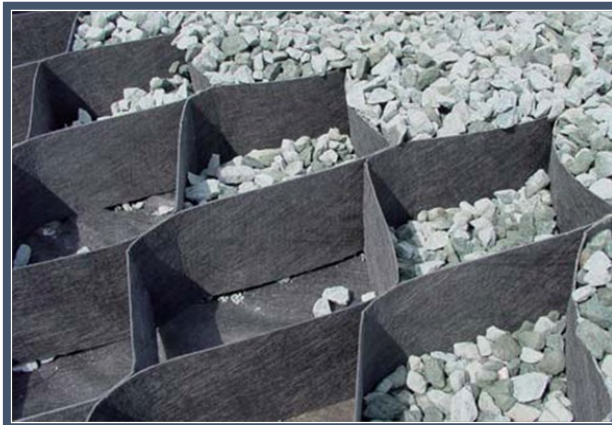
Figure 12 Examples of Cellweb filling with angular stone
