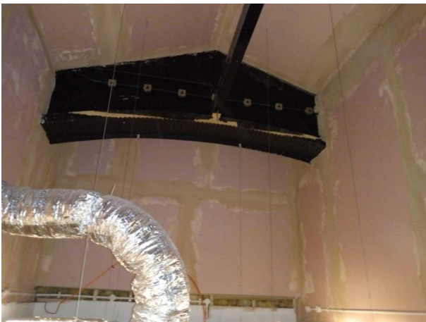
Void structure, northern section of pitched roof.
