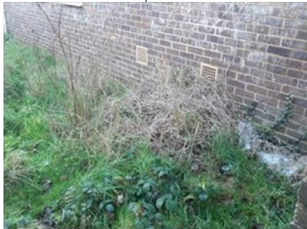
TN4 Pile of vegetative material beside the eastern wall of B1.
