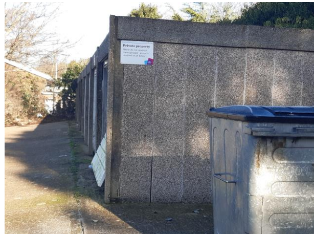
Garages along the south-eastern survey area boundary.
