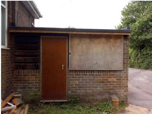
Northern extension, storage room
