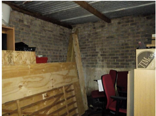
Interior of northern extension
