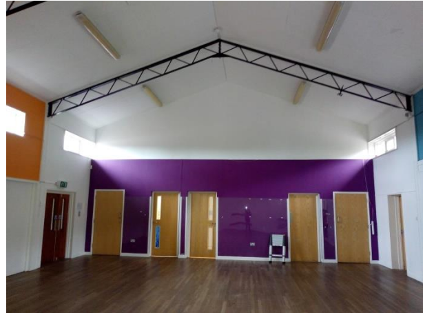
Vaulted roof in main hall.
