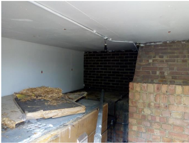
Water tank room
