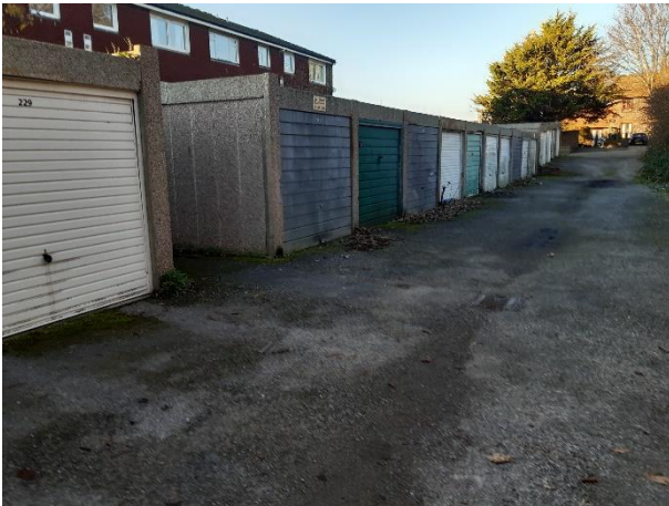
Garages along the western survey area boundary.
