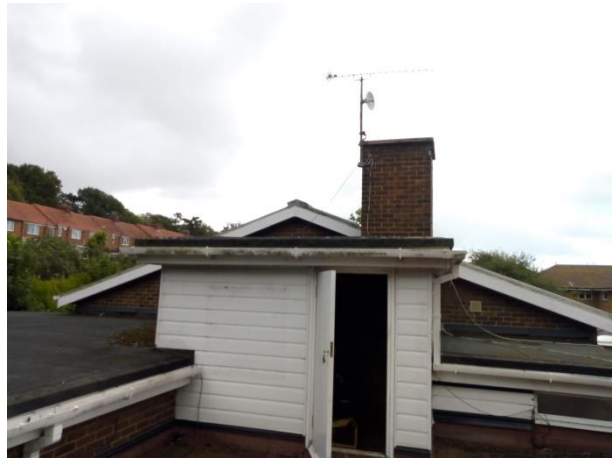
External view of water tank room
