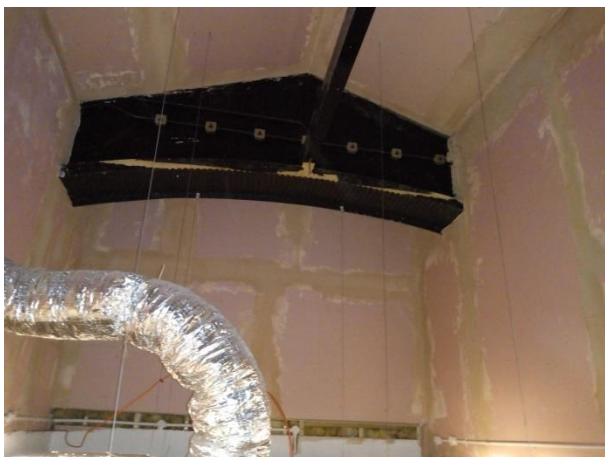
Void structure, northern section of pitched roof
