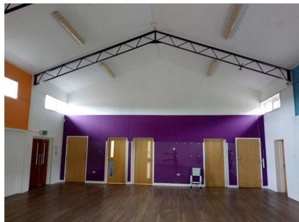
Vaulted roof in main hall
