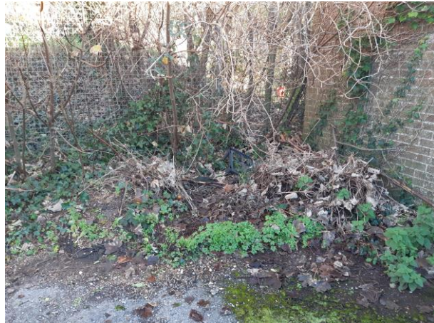
TN6 Piles of rubble and vegetative material on hardstanding in the south-western corner of the survey area.
