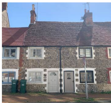
18th-Century. 44-50 High St Cottages built using flint and red brick, are listed buildings and face the old brewery
