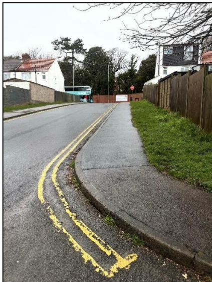
Photograph 5: Existing conditions along Locks Crescent
