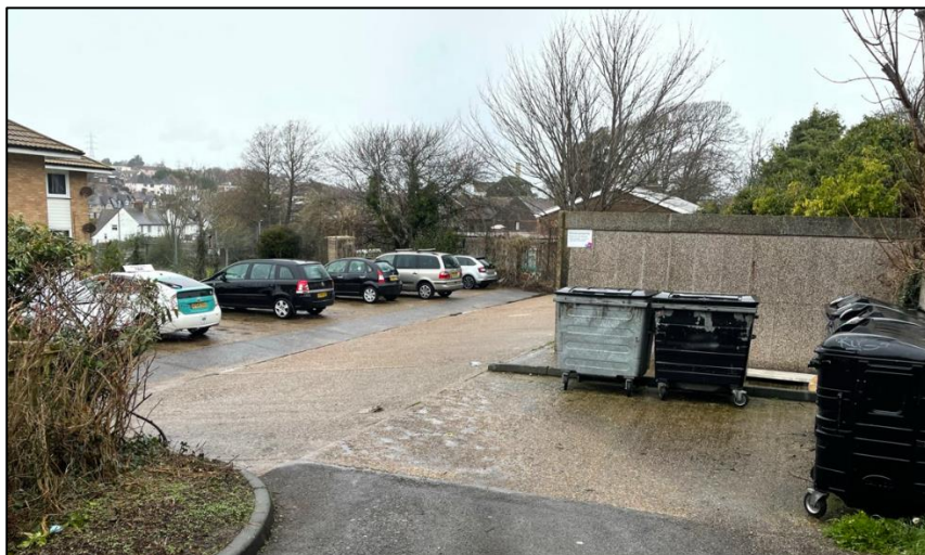
Photograph 7: Blakers Close Parking Area
