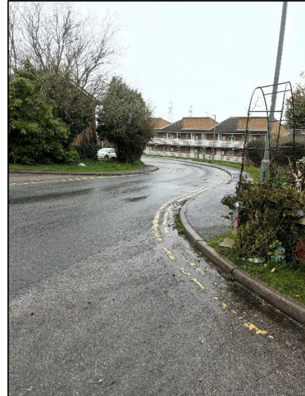
Photograph 6: Existing conditions along Locks Crescent
