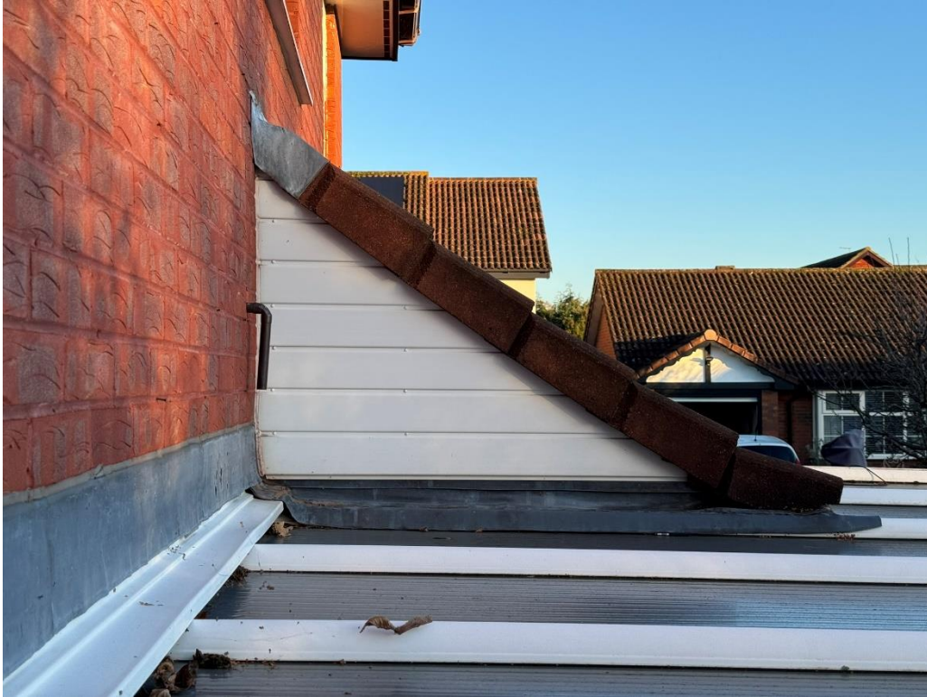
Plate 7. PVC cladding at western end of pent-roof section.
