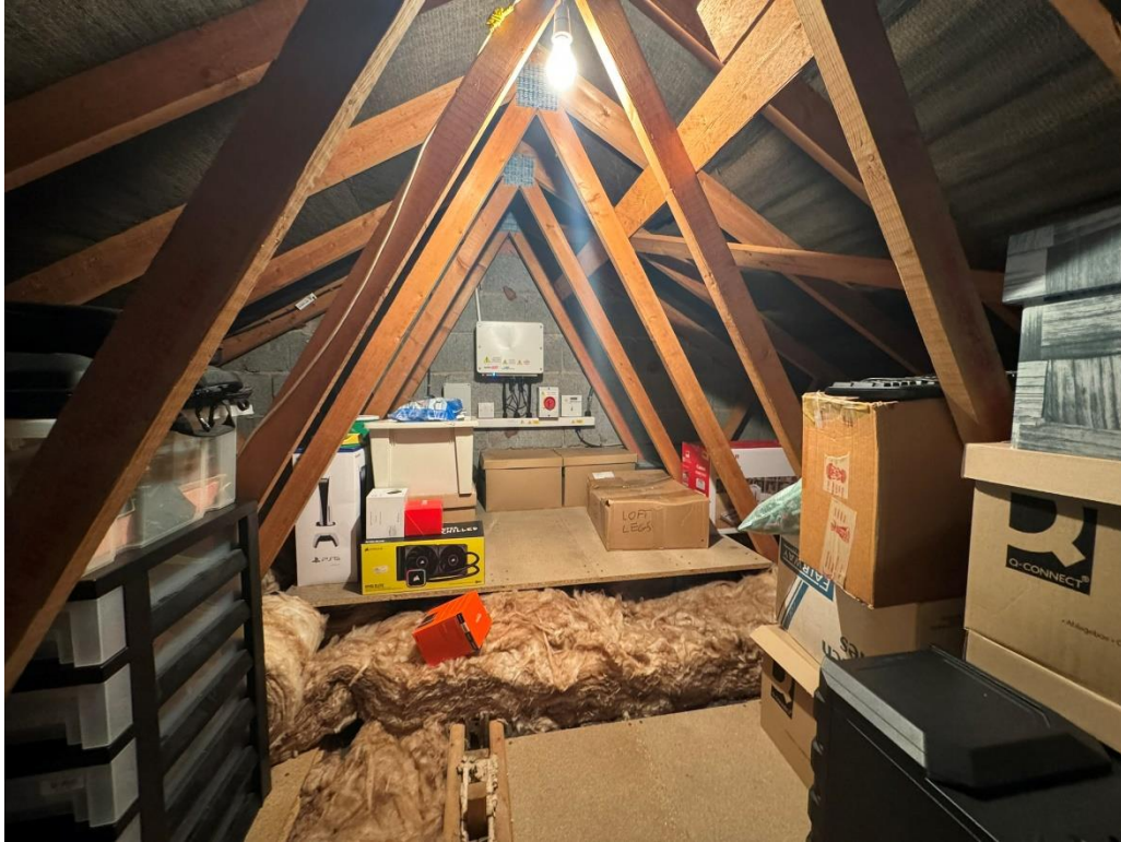
Plate 9. Roof void, looking towards western gable.
