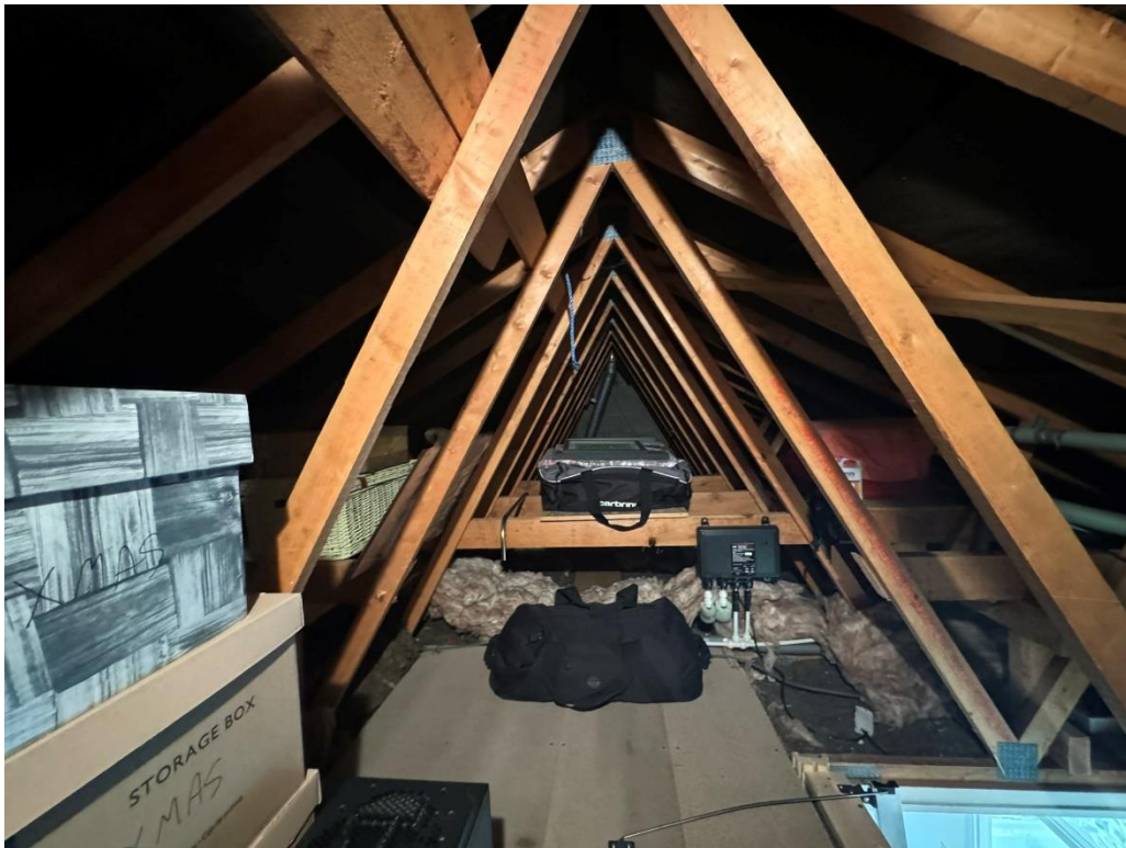
Plate 10. Roof void, looking towards eastern gable.
