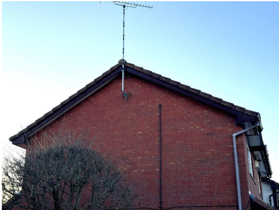
Plate 2. Eastern gable end.
