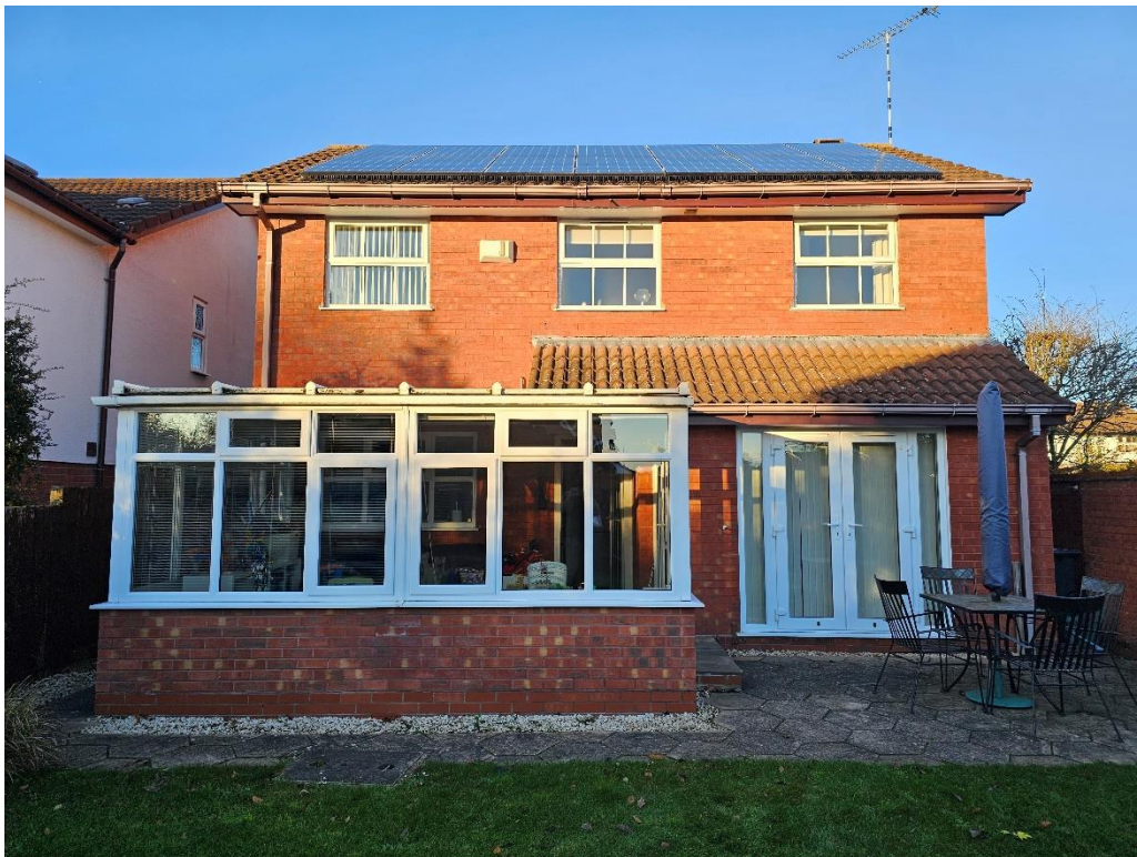
Plate 4. Southern aspect, showing the conservatory and pent-roofed section to be removed.
