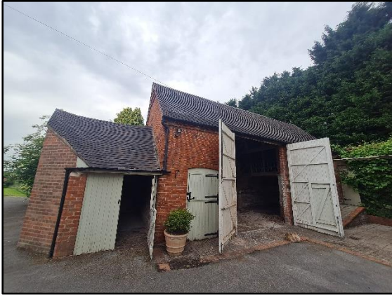
Plate 1: showing a typical external view of the Barn (B1). Photograph looking north.
