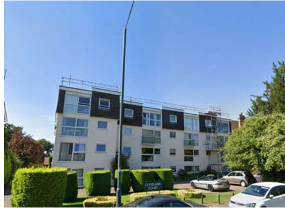
Apartments 60's non vernacular development
