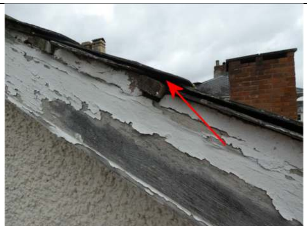
Photograph 12. Opening under a slate above the west gable on the central part of the house
