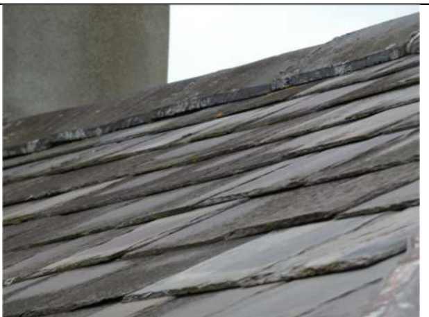
Photograph 10. Example of the slates on the central part of the house
