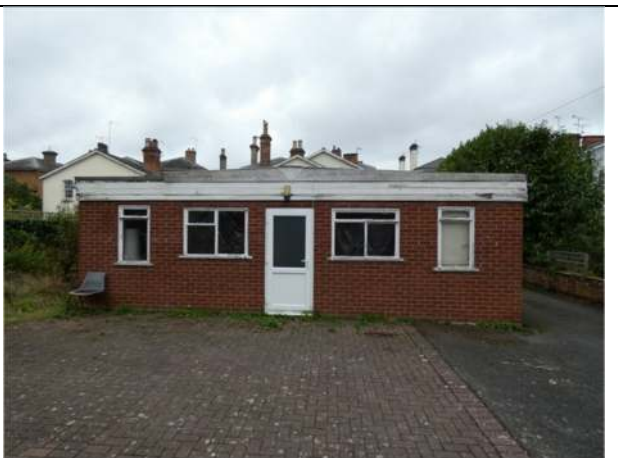
Photograph 6. The east elevation of the eastern part of the house
