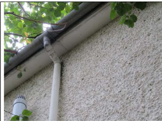
Photograph 17. Example of the soffit on the main part of the house
