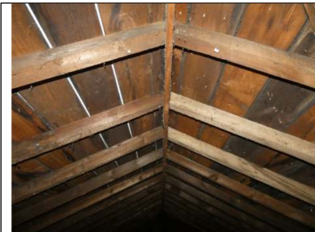
Photograph 21. Sarking and roof timbers within the main part of the house
