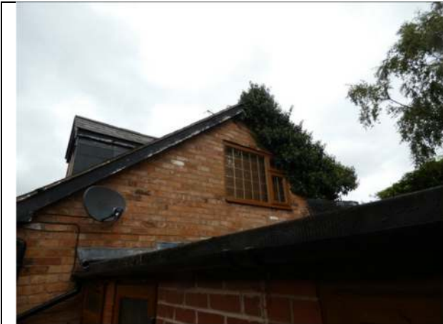
Photograph 25. The south elevation of the cottage
