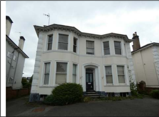
Photograph 1. The west elevation of the house
