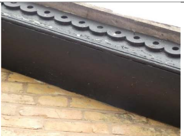
Photograph 30. Further example of sealed soffits on the cottage
