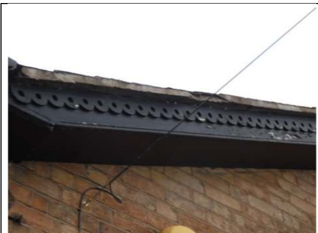
Photograph 29. Example of sealed soffits on the cottage
