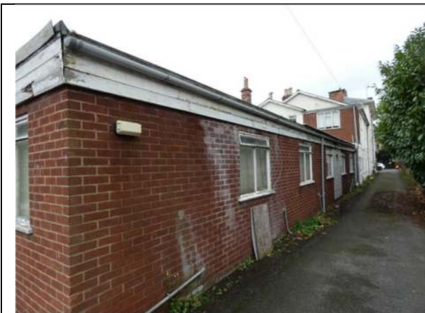
Photograph 5. The north elevation of the eastern part of the house
