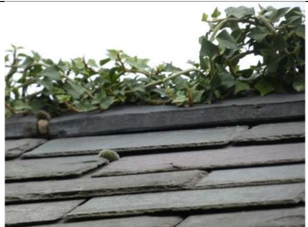
Photograph 26. Example of the slates on the roof of the cottage
