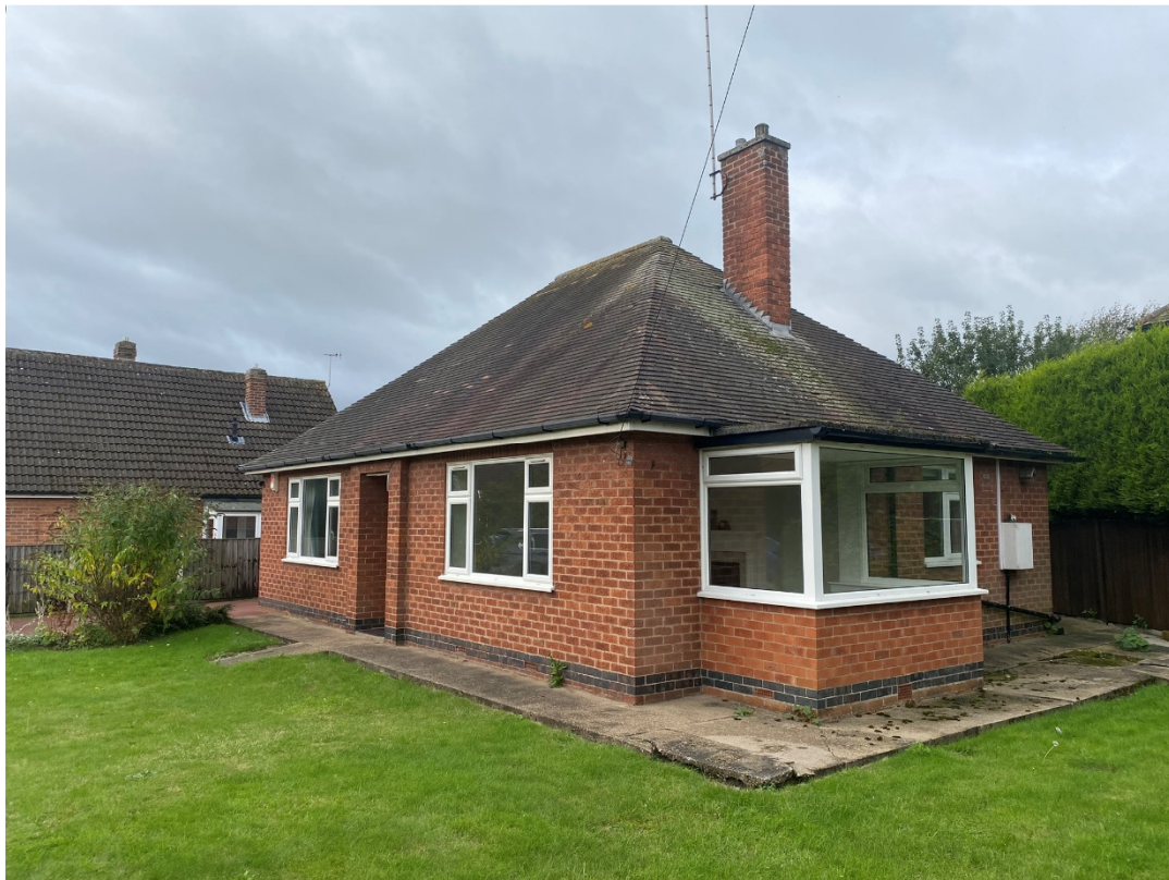
Existing front and side view of No 53 College Street, East Bridgford
