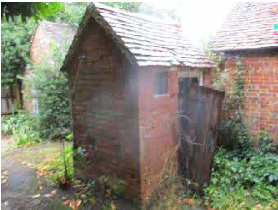
Old outside toilets
