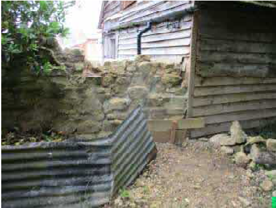
Boundary being rebuilt
