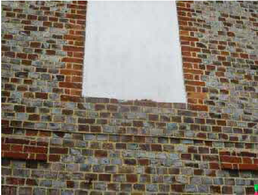
Ply panel to window opening
