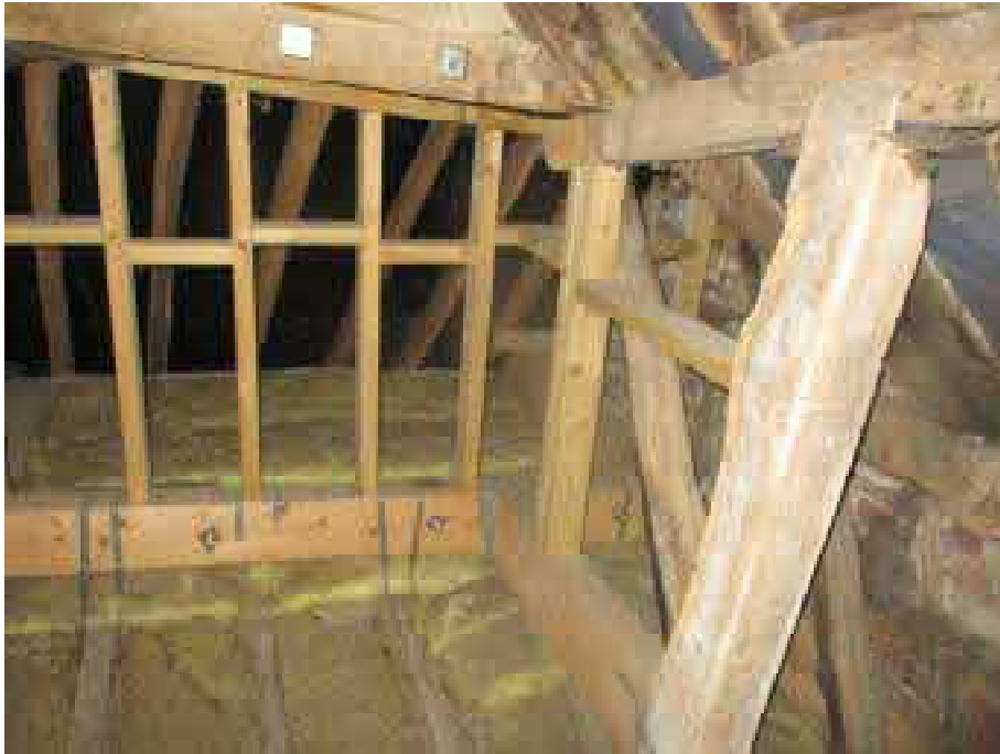
Rear roof void
