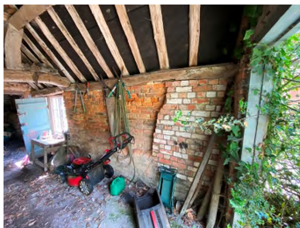
Figure 9: Brick construction of the western side of the south wall
