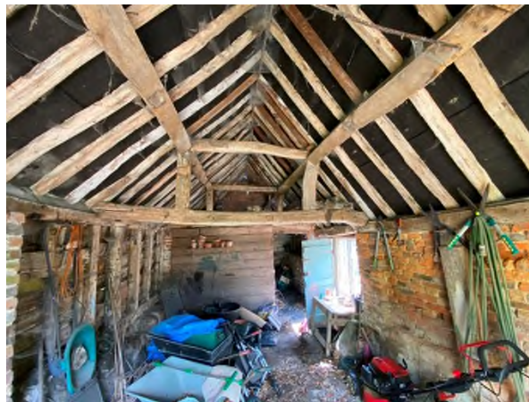
Figure 8: Interior of the garage looking east
