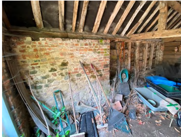
Figure 10: Mixed brick and rubble stone with stud frame over a plinth on the northern side of the garage
