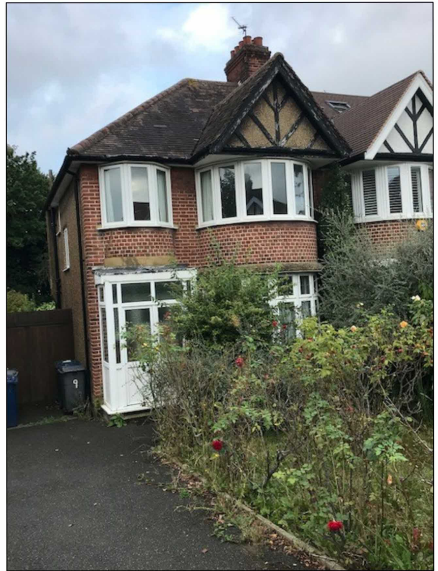
FRONT VIEW OF No 9 MAXWELTON CLOSE (Looking W).
