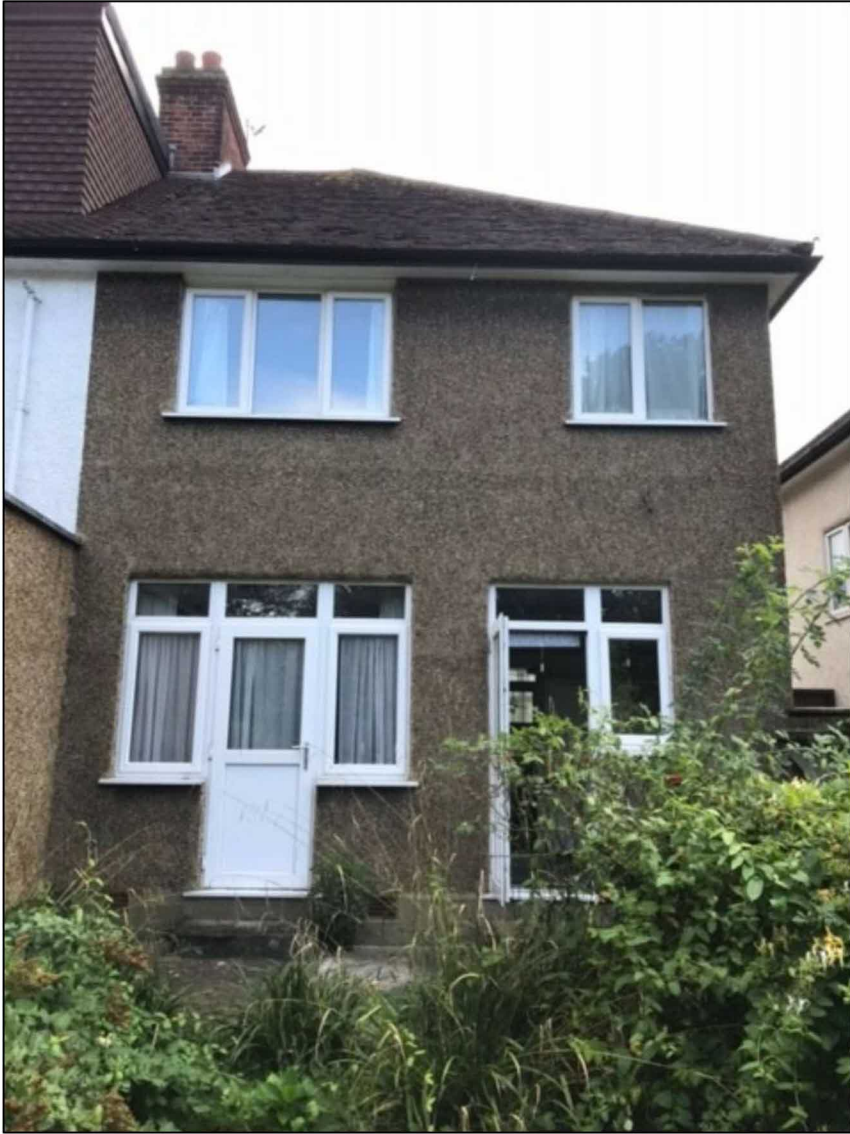
REAR VIEW OF No 9 MAXWELTON CLOSE (Looking East).
