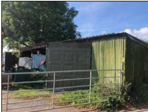
Photograph 3: The eastern Site boundary. Photograph showing building B1A on the right-hand side and building B2 on the left-hand side.
