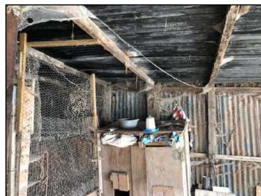
Photograph 10: The internal aspects of building 3. Photograph taken looking east.
