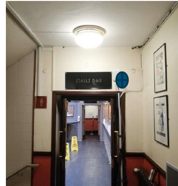
Location AP 13 - Ground Floor/ Stalls Level - adjacent to existing cable routes
