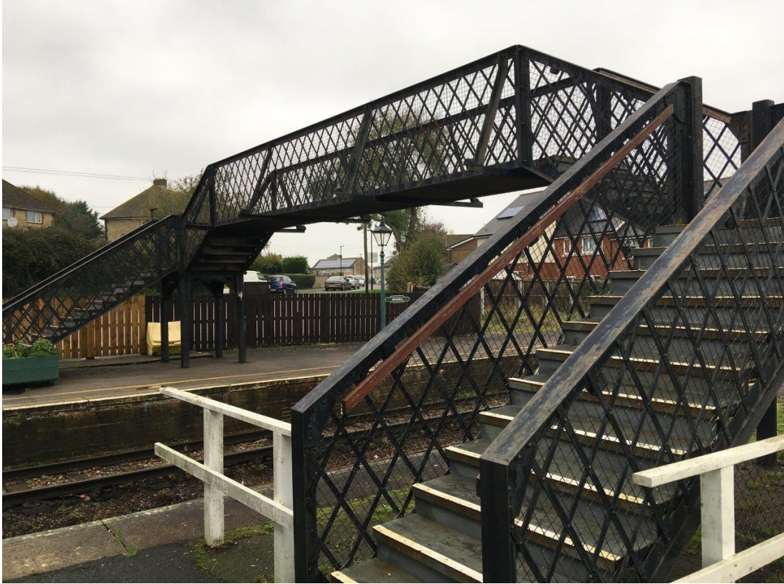
Figure 2 - Photograph of Brading Footbridge
