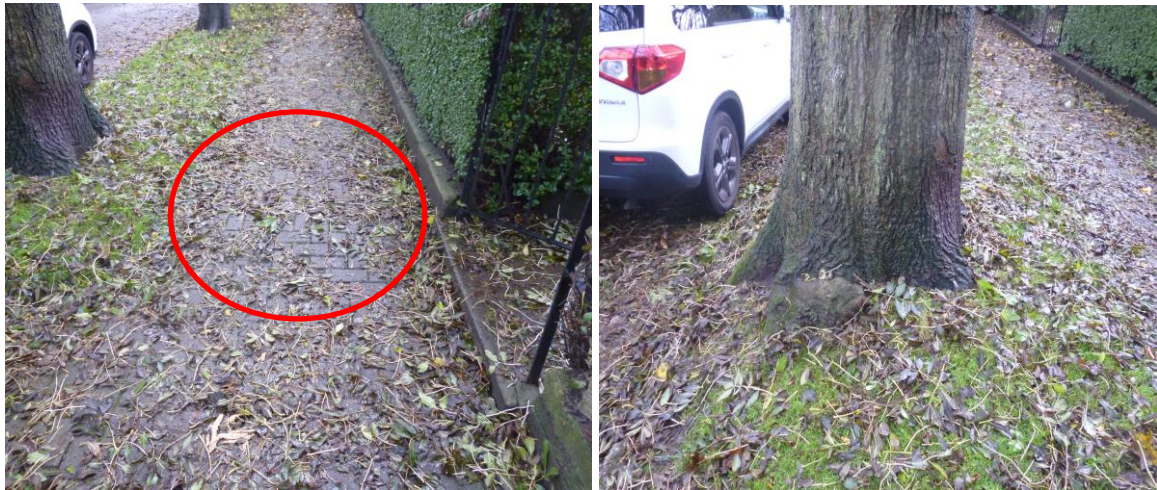
Photograph 5a to e – The pavement and highway at the base of T1 (signs of lifting to the pavement).
