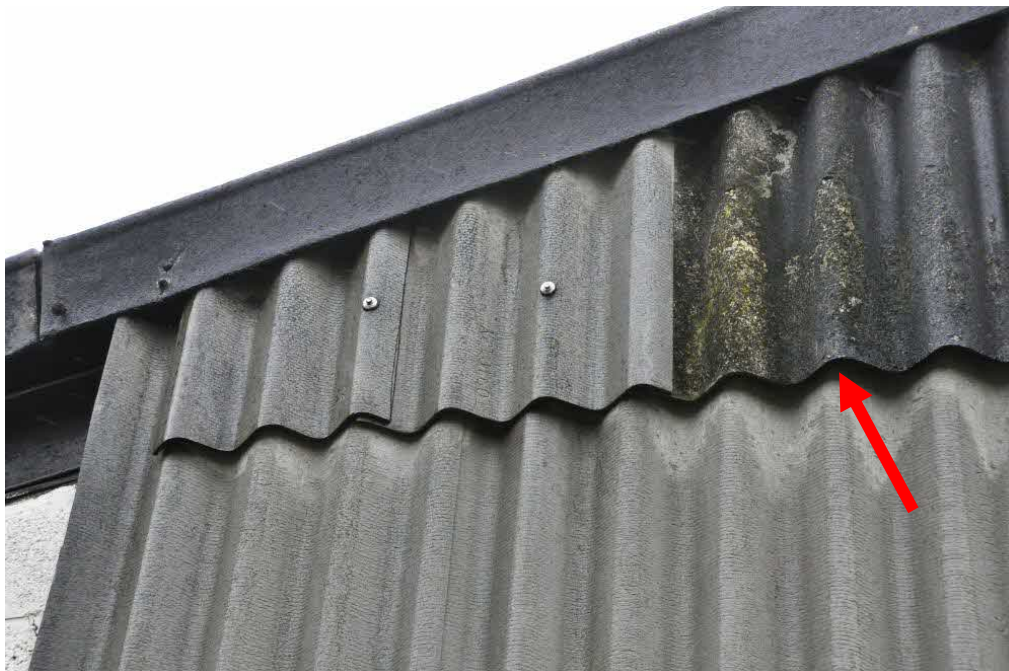
View of overlapping external sheet walls. The overlap creates a small dark cavity with low potential for use by bats
