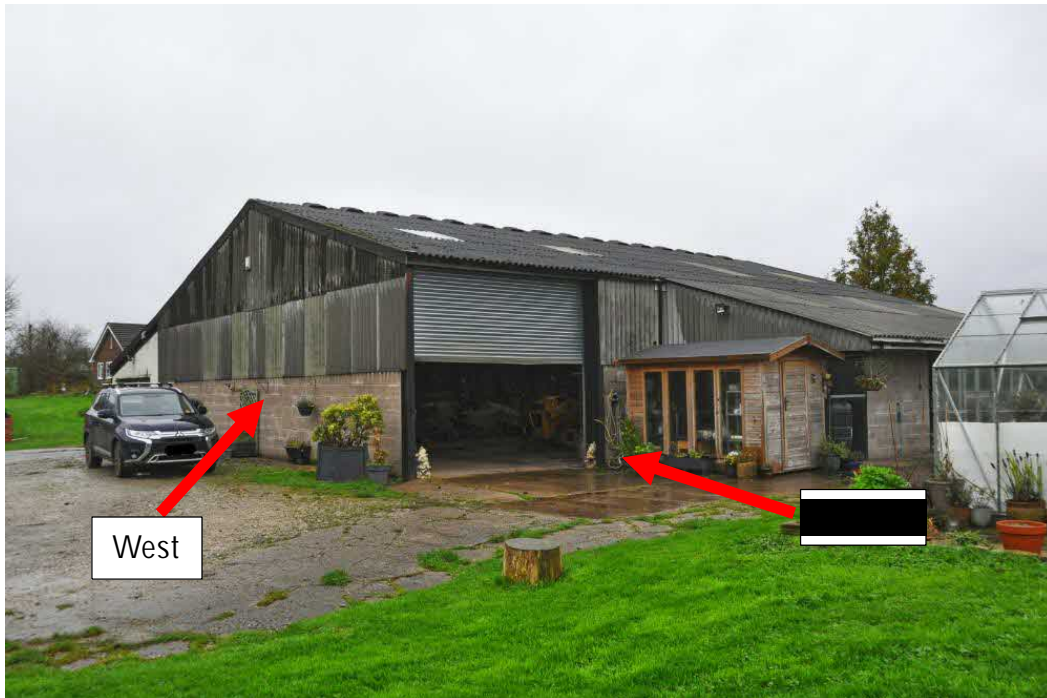
View of the barn building showing west and south elevation
