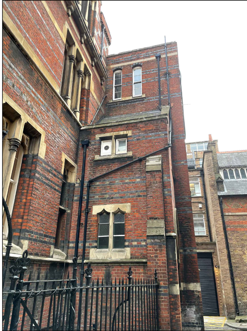
Photo 2: North Elevation to be extended for lift shaft
