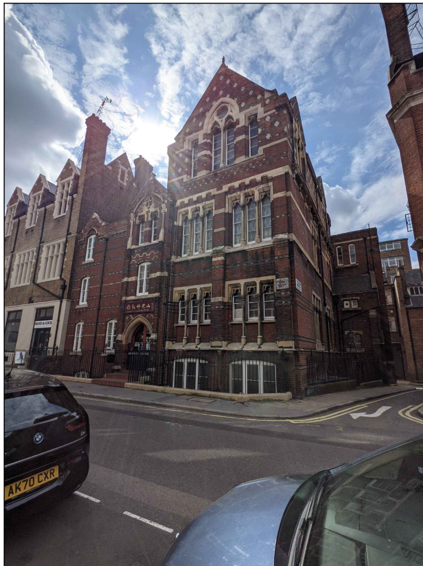
Photo 4: View looking South to North Elevation and side elevation
