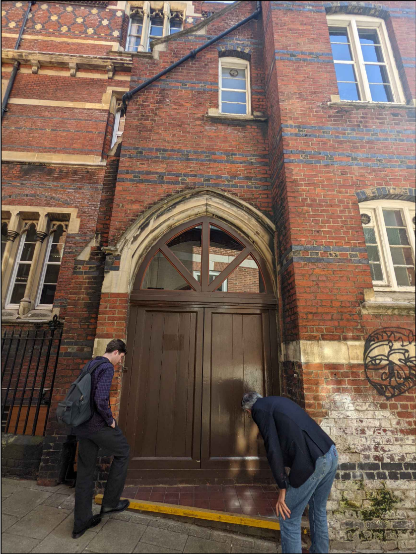
Photo 1: Door GF D17
