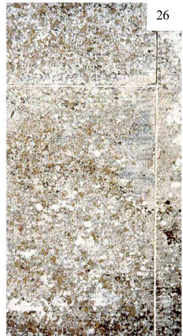
26. The filled joint after removal of adhesive tape.
