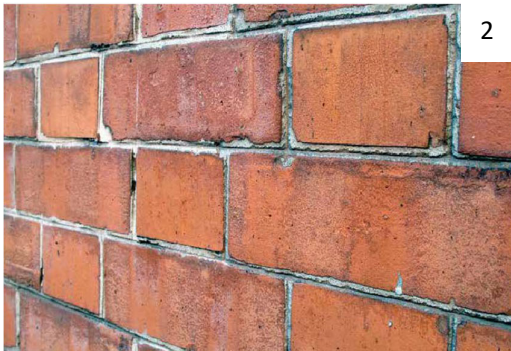
2. The mortar is incised so a groove runs through the centre of the joint. This is called penny round or struck pointing.
