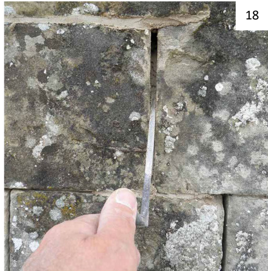
18. Using tools that match the width of the joint allows the mortar to be compacted ensuring a fully filled joint.
