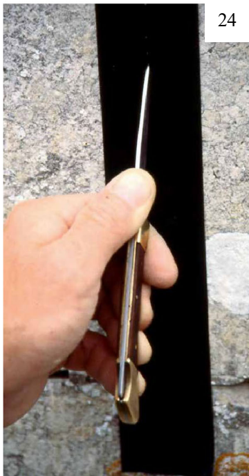
24. Incision of the tape through the joint.
