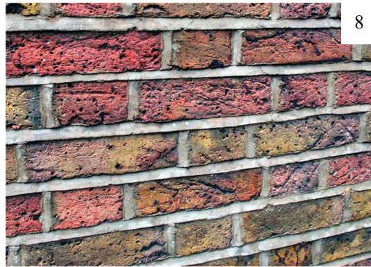
8. Ribbon or strap pointing to brickwork. A style similar to weather-struck being proud of the masonry and smoothed off. Often used to give a regular joint width to irregular brick and stone masonry.
