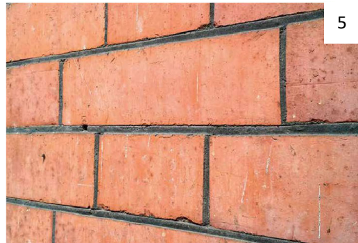
5. This joint has been indented to form a V-shaped groove which is referred to as keyed pointing.
