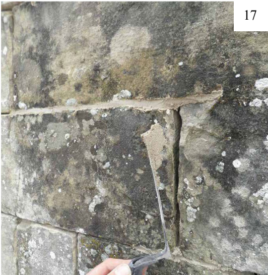
17. A wedge of mortar being inserted into the joint with a pointing iron.
