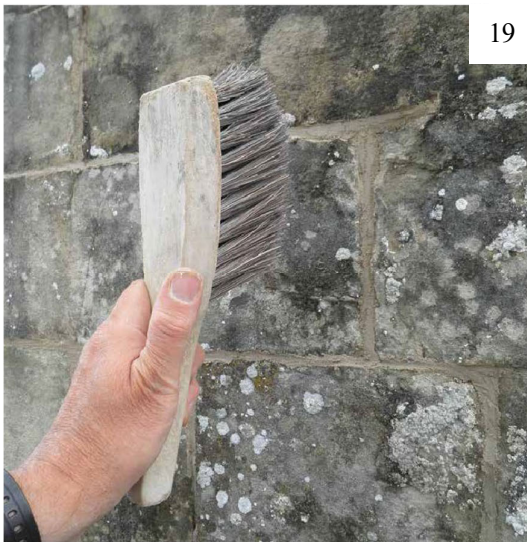
19. The mortar being hit with a stiff bristled chum brush to compact the mortar, remove laitance and expose the aggregate.
