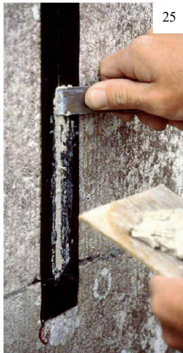
25. Pressing mortar into the joint using a pointing iron.
