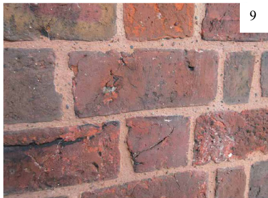
9. Example of good repointing
