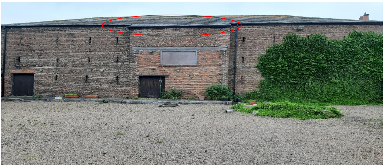
Plate 4.1 – the neighbouring barn; NE of the project where a Common pipistrelle roost is present. Highlighted is the areas bats were emerging from
