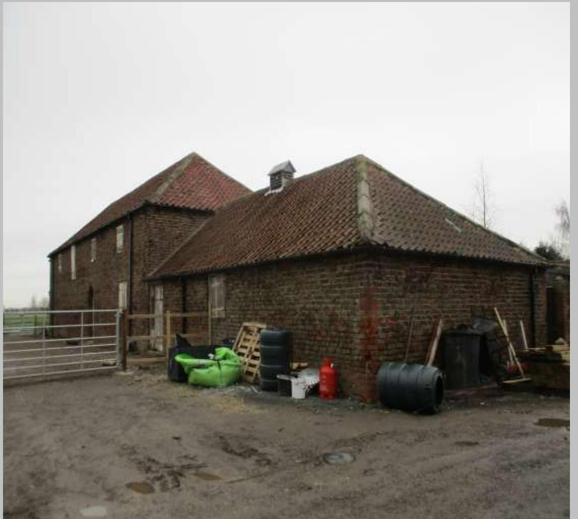
SOUTH VIEW : EXISTING SINGLE STOREY STORAGE BARN TO BE CONVERTED.
