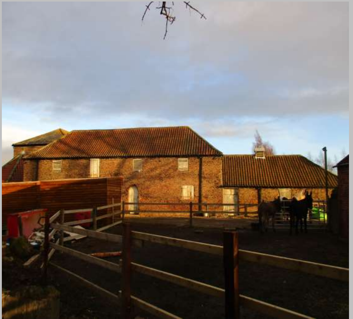
WEST VIEW : EXISTING TWO STOREY STORAGE BARN TO BE CONVERTED.
