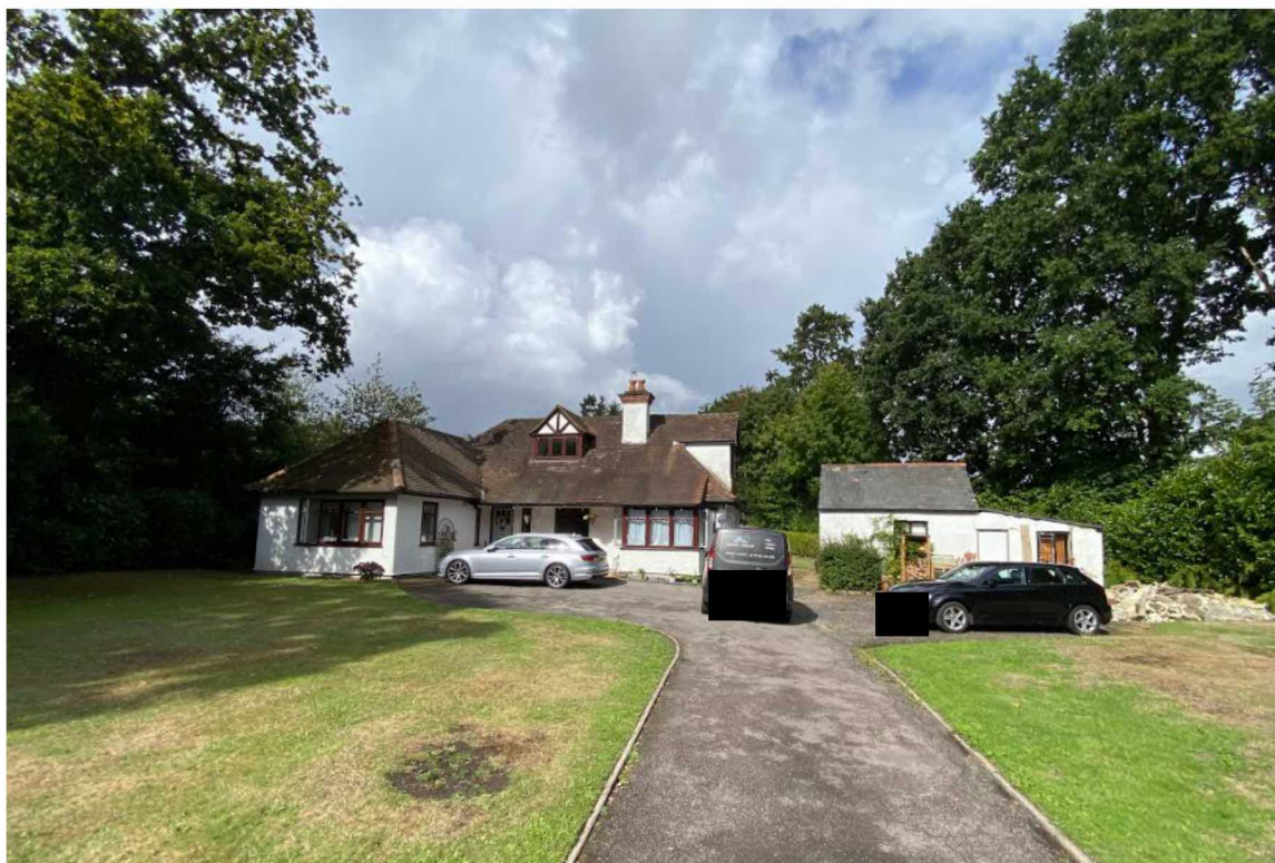
Photographic plate showing existing dwelling and hard landscape
