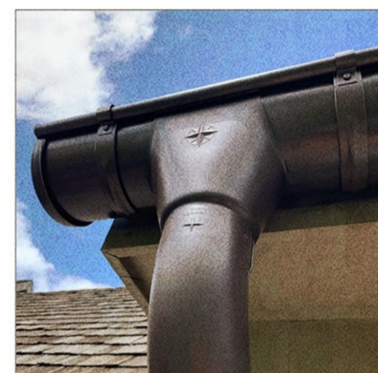
GUTTERING Half round black coated galvanized steel gutters and downpipes
