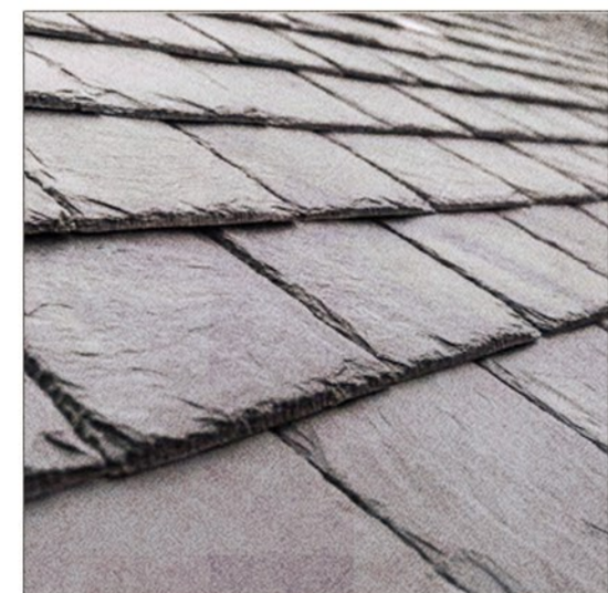
ROOF Tiles/ Slates
