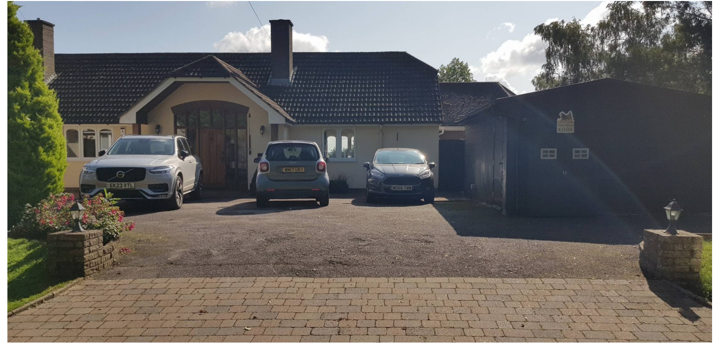
Fig 18. EXISTING DRIVE Parking and outbuildings
