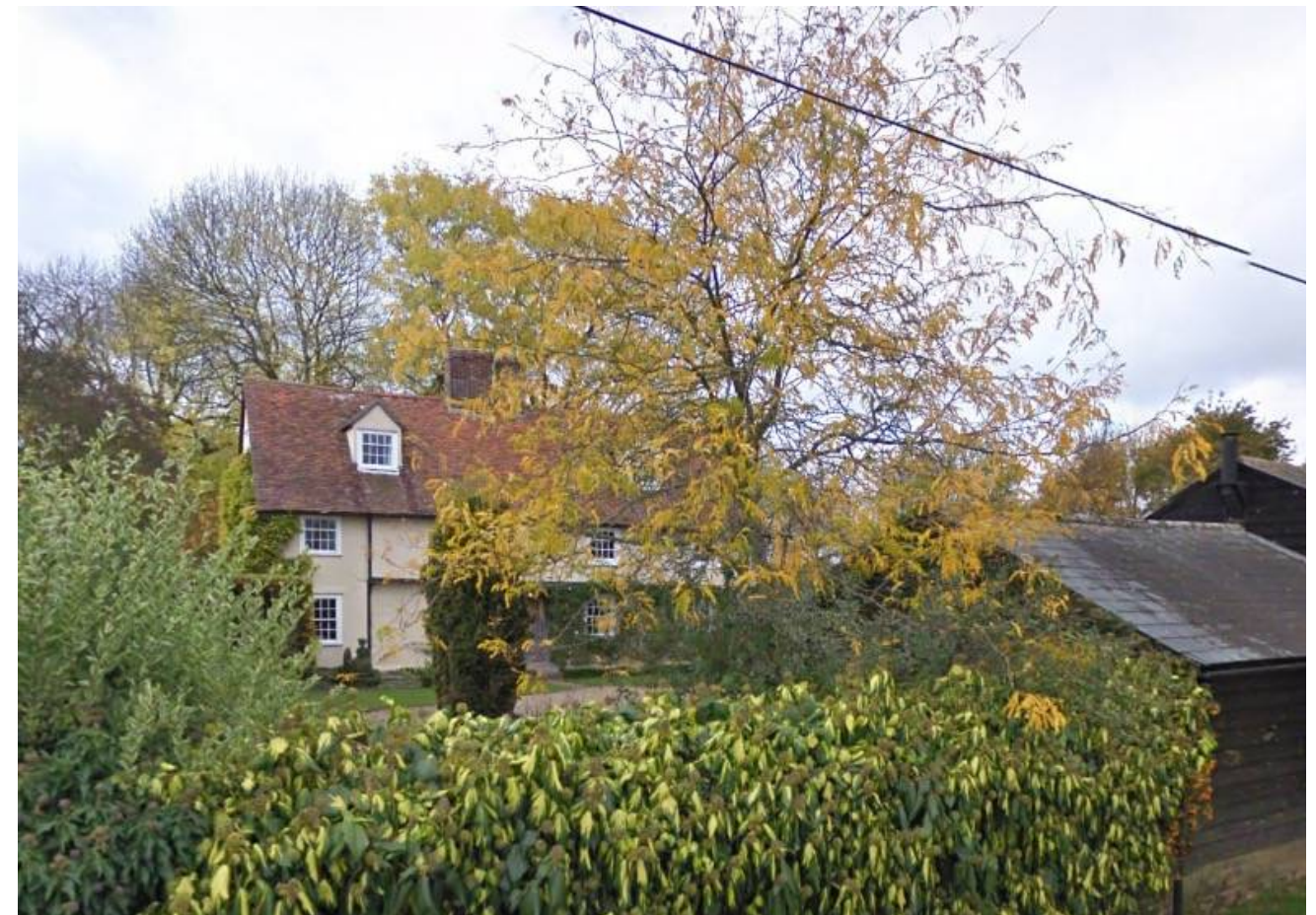
Fig 6. KENNEL FARM FARMHOUSE – East Elevation
