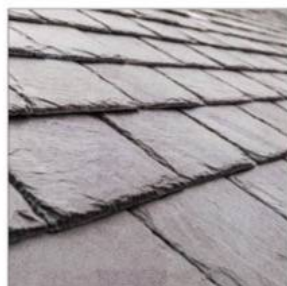
ROOF Tiles/ Slates
