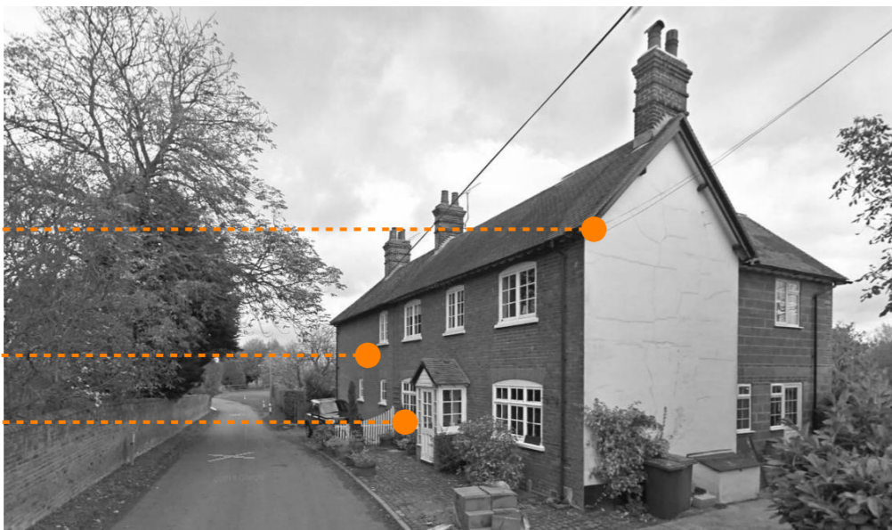
Fig 46. PIGGOTS COTTAGES – 2 storey
