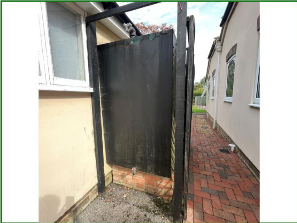
Photo No.15: Shows an oil tank atop a brick plinth between the house and garage and facing north.
