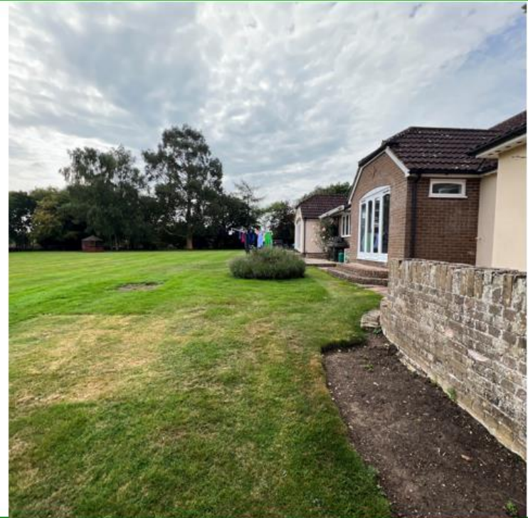
Photo No.12: Facing south across the eastern face of the property showing lawns and soft landscaping.
