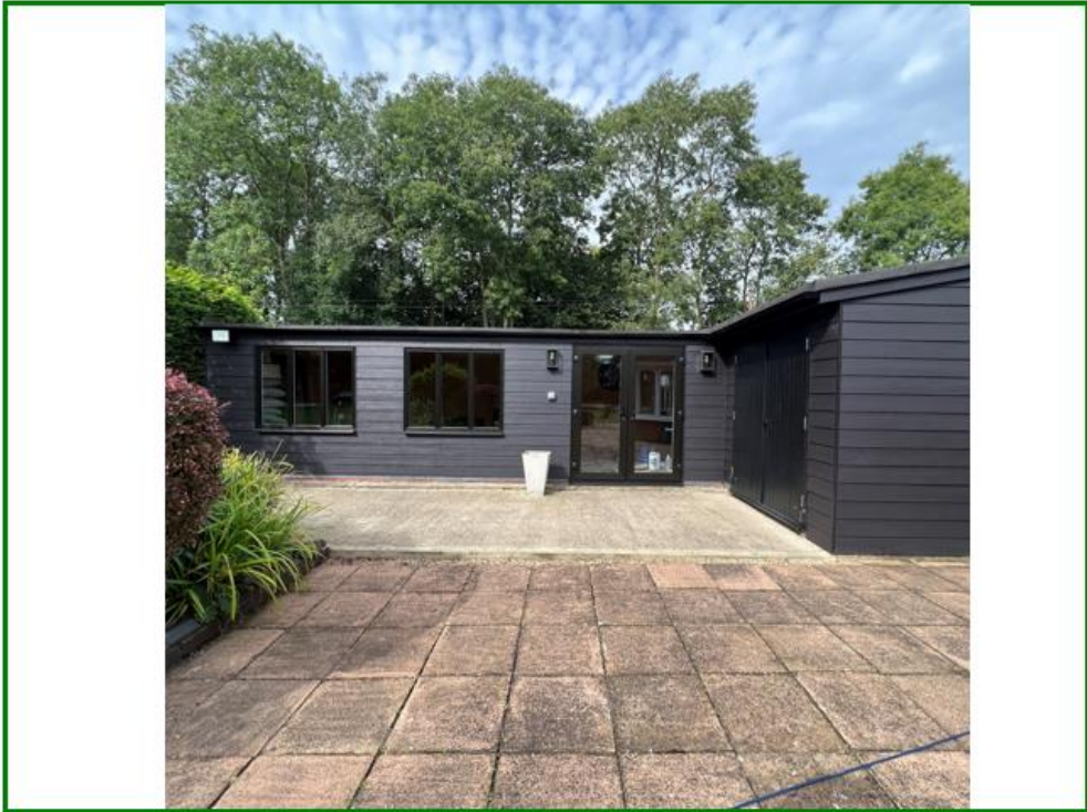
Photo No.18: Shows the outbuilding to the southwest of the main house facing slightly northwest.
